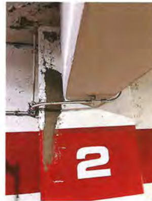
Photo 18: Typical completed concrete test pit patching prior to painting
