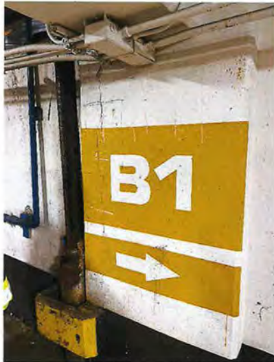
Photo 1: Column on Level B at D/13
