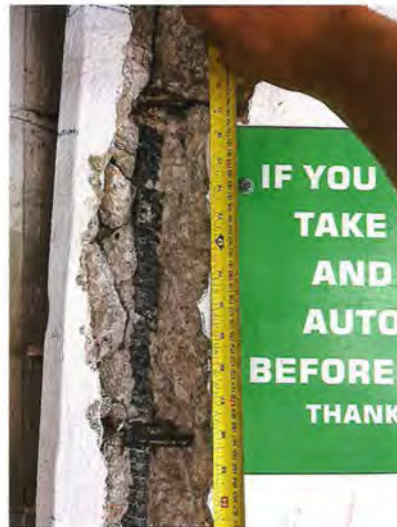
Photo 12: Column on Level P3 at D/3
