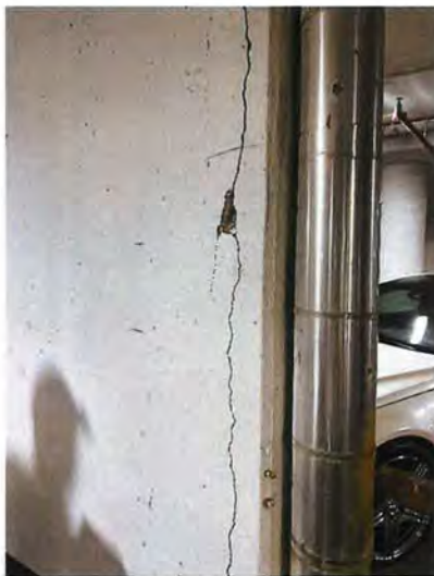
Photo 3: Edge of Wall on Level P1 at D/28
