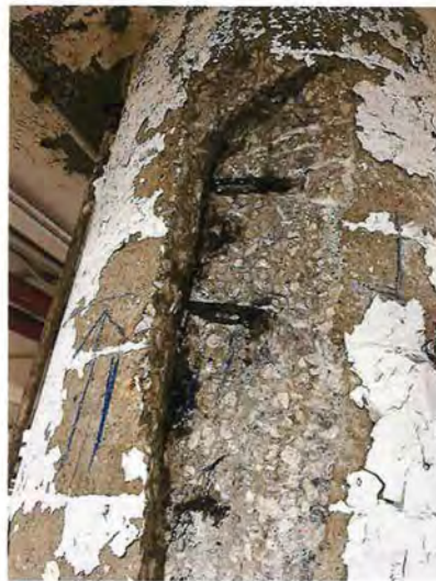
Photo 10: Column on Level P1 at D/34
