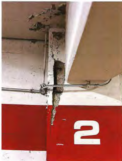
Photo 11: Column on Level P2 at G/17
