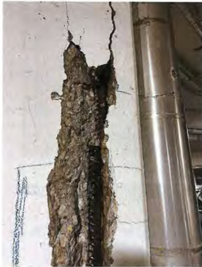
Photo 9: Edge of Wall on Level P1 at D/28
