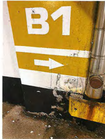
Photo 2: Column on Level P1 at D/17
