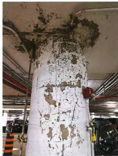
Photo 4: Column on Level P1 at D/34
