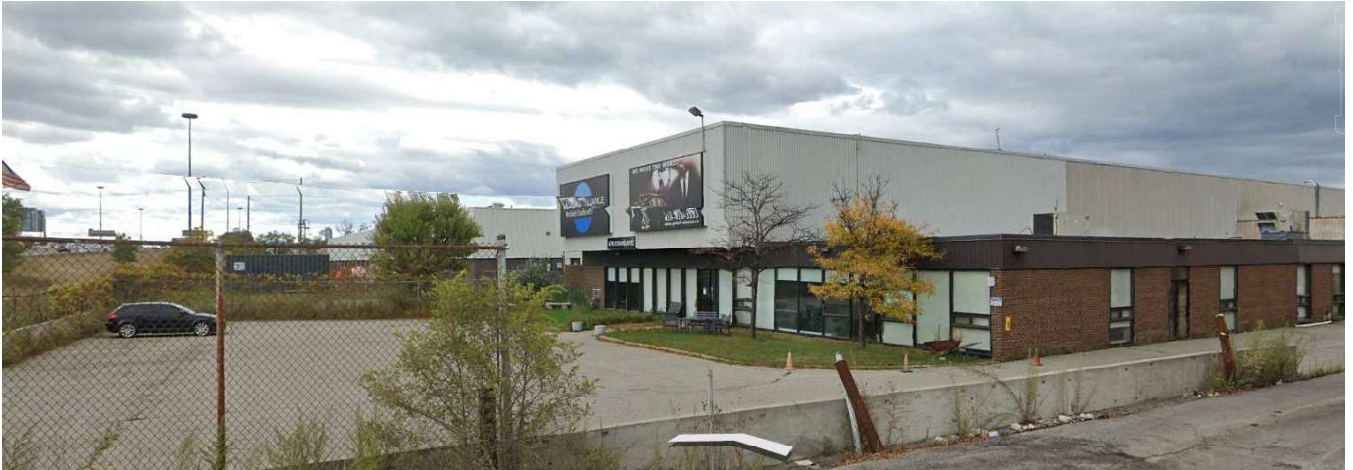
View of subject premises, facing east
