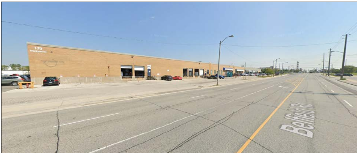
Figure 3: Looking Northwest from Belfield Road towards 170 Brockport Drive
