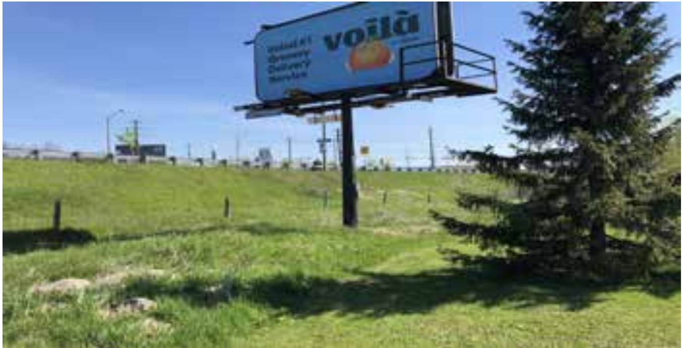
Plate 2. Existing sign to be removed.
