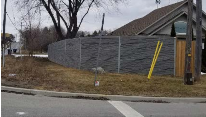
Attachment 2: Picture of stone fence on flankage yard
