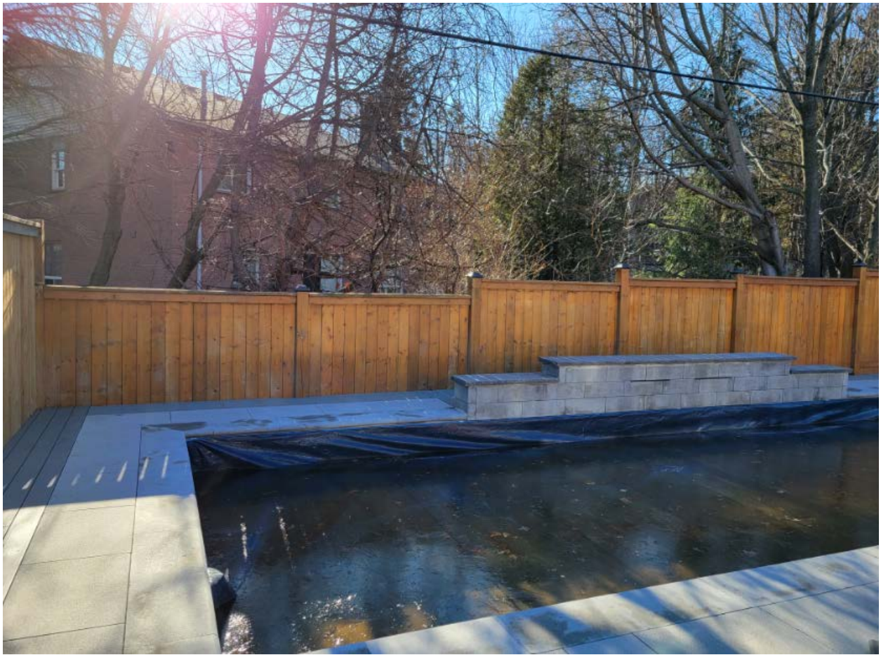
Attachment 3 – Photo of south property line fence
