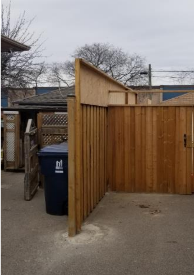
Attachment 2: Photo of fence from driveway
