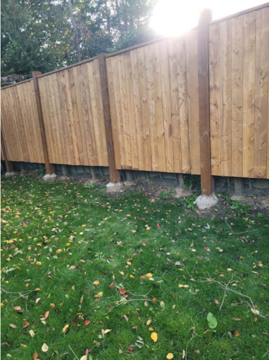
Attachment 3: Photo of fence on west side of property
