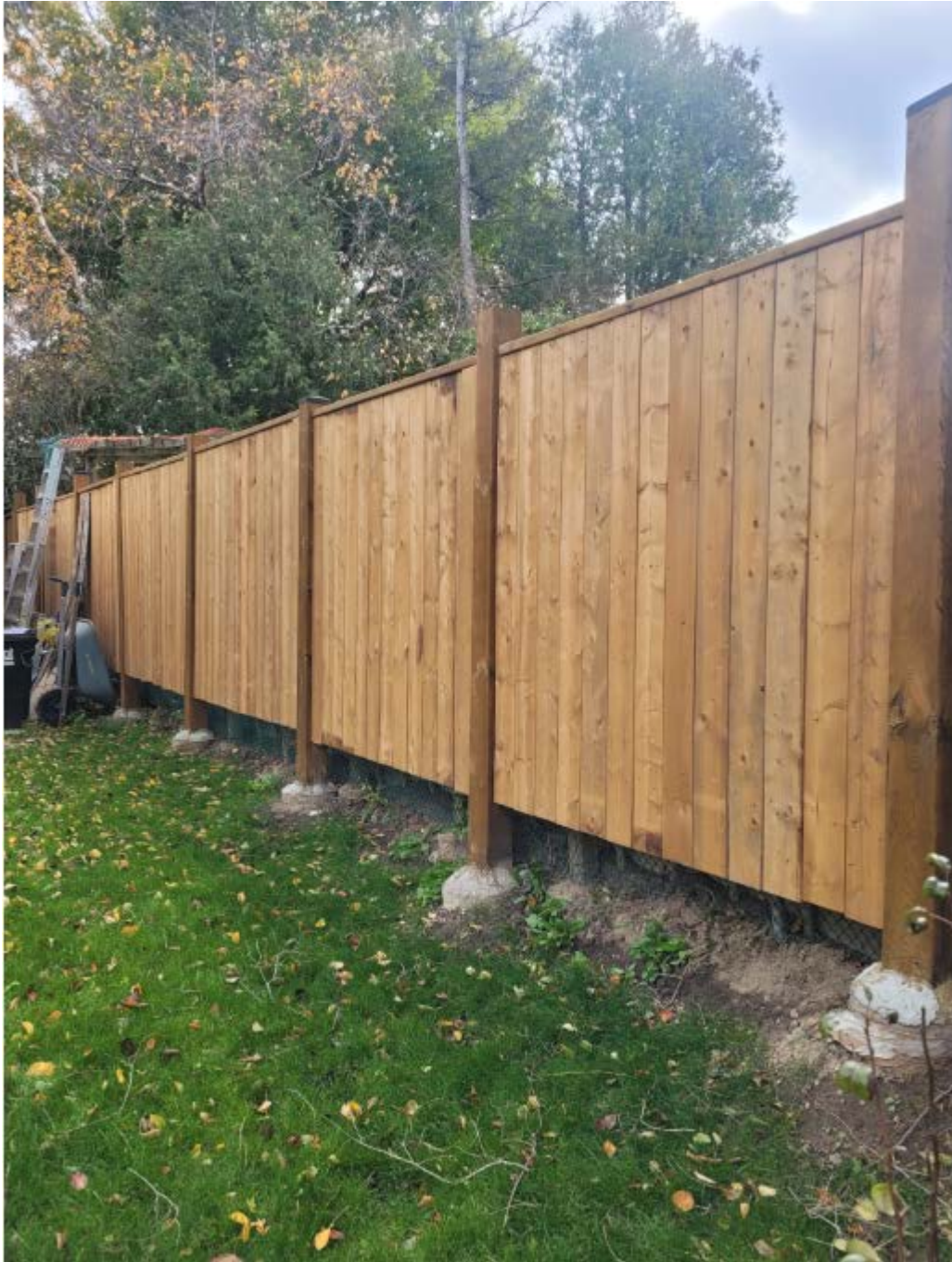
Attachment 2: Photo of fence on west side of property
