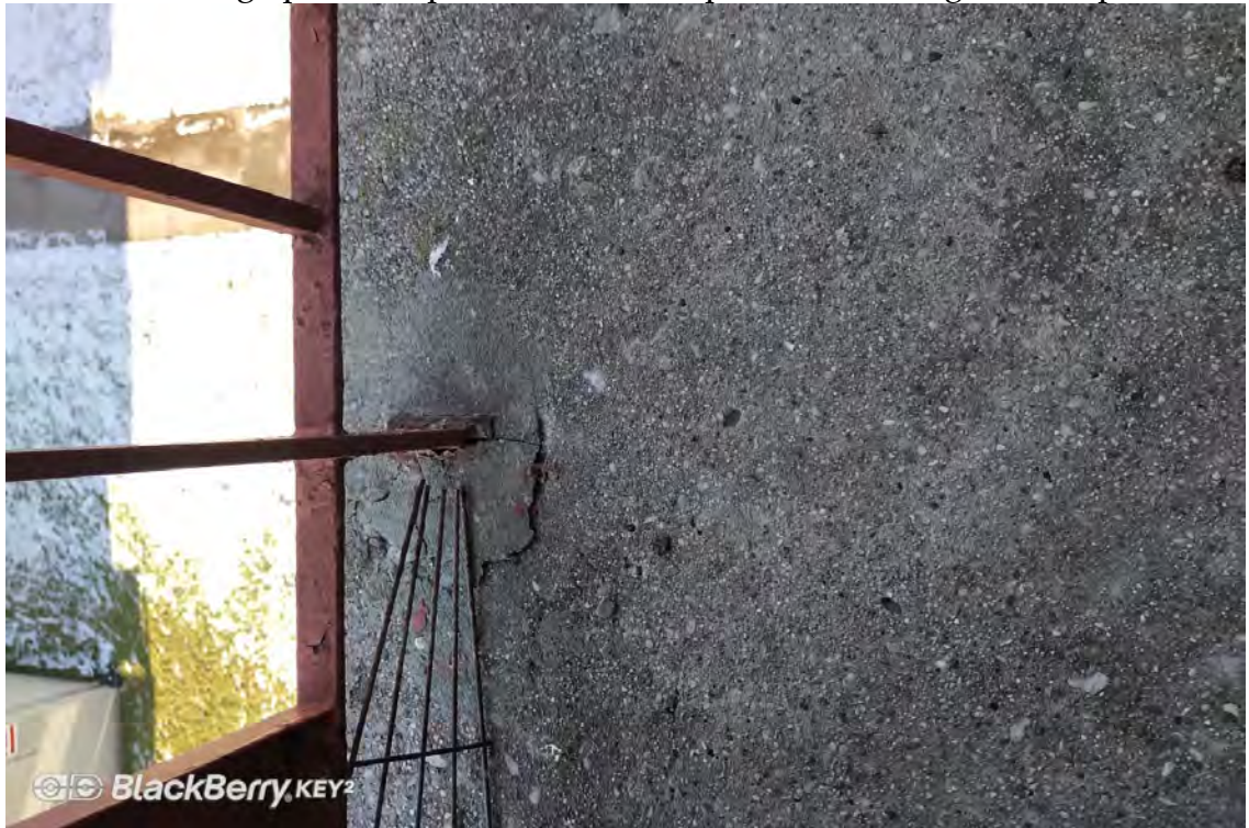
Photo No. 8: Another location with spalling concrete around guardrail post
