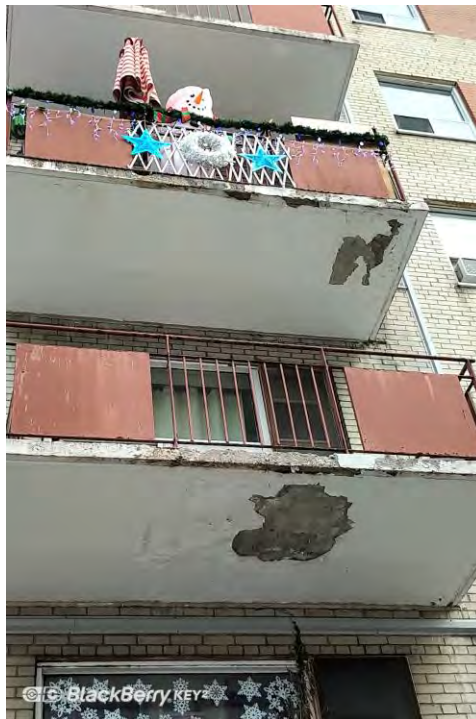
Photo No. 14: Concrete delaminations at balcony slabs edges and soffit
