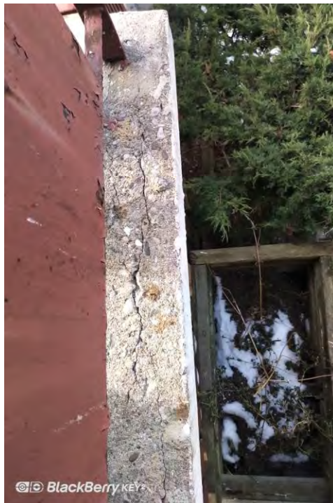
Photo No. 10: A heavily cracked balcony slab front edge
