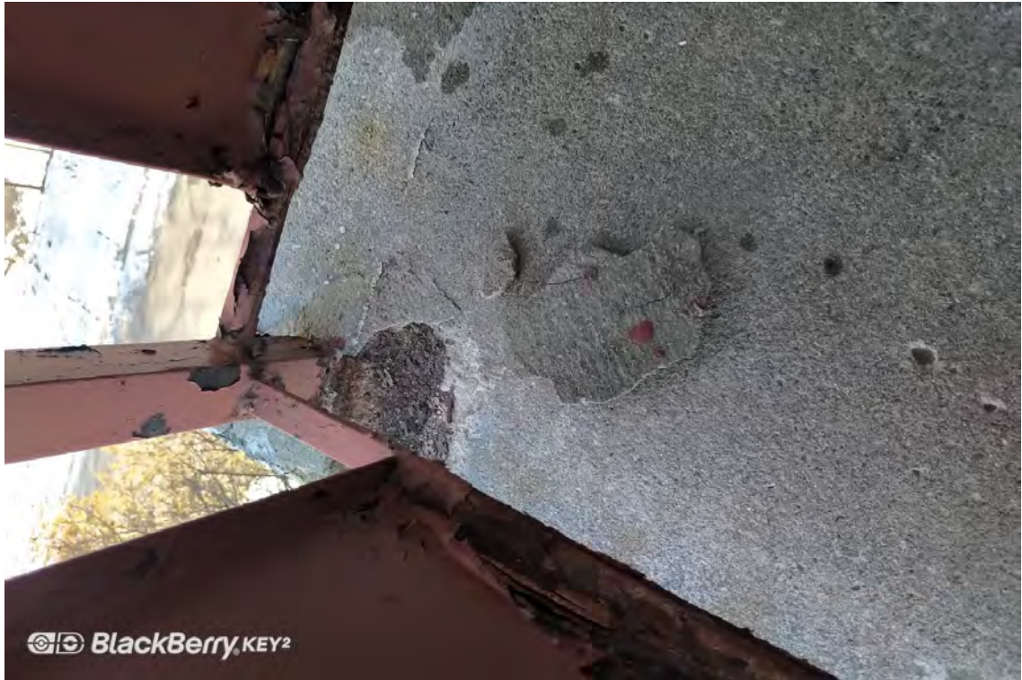
Photo No. 7: A large piece of spalled concrete separated from a guardrail post location
