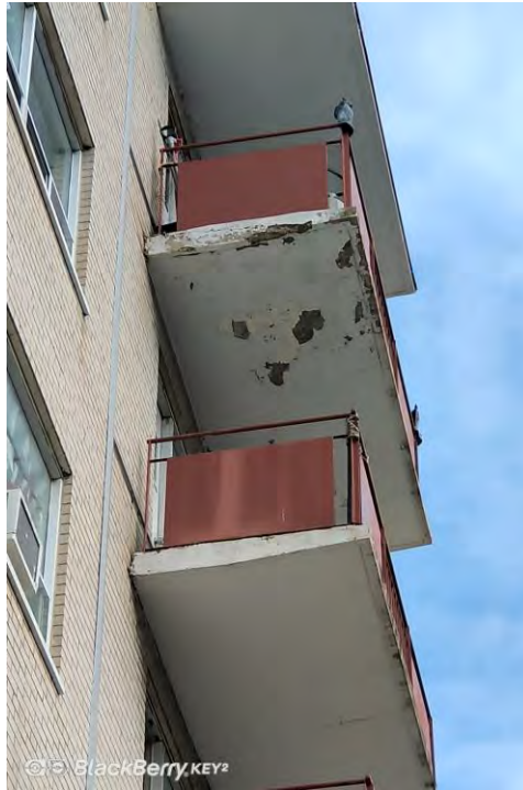
Photo No. 13: Concrete delaminations at balcony slabs edges and soffit
