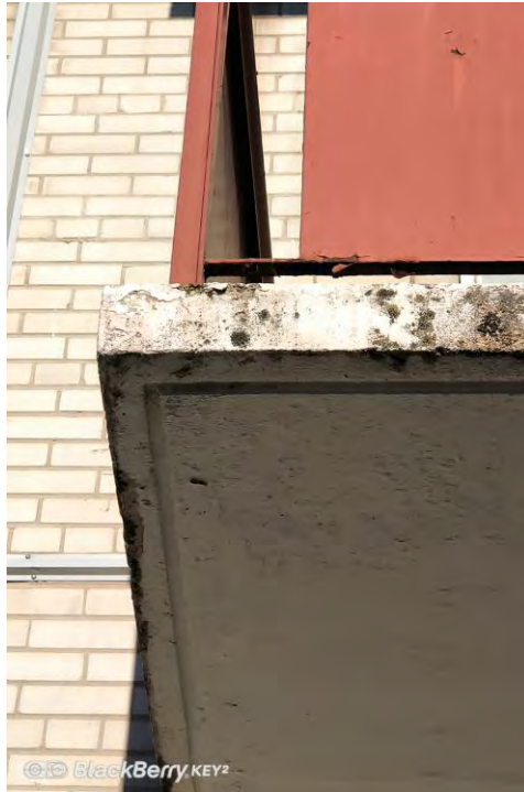
Photo No. 3: A heavily cracked slab edge
