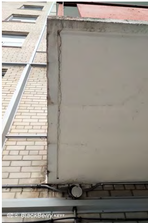
Photo No. 12: A heavily cracked balcony slab side edge
