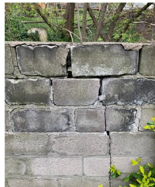
Figures 2,3, 4. Views showing retaining wall deterioration.
