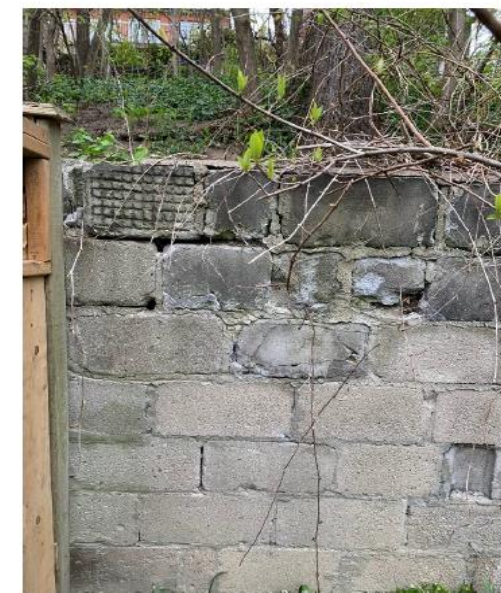
Figures 2,3, 4. Views showing retaining wall deterioration.
