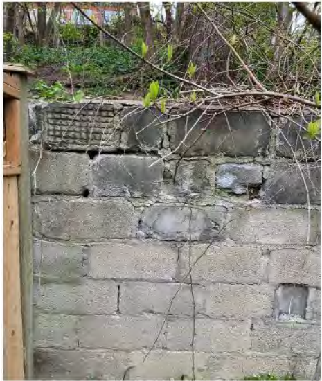
Figures 2,3, 4. Views showing retaining wall deterioration.
