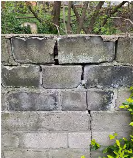
Figures 2,3, 4. Views showing retaining wall deterioration.
