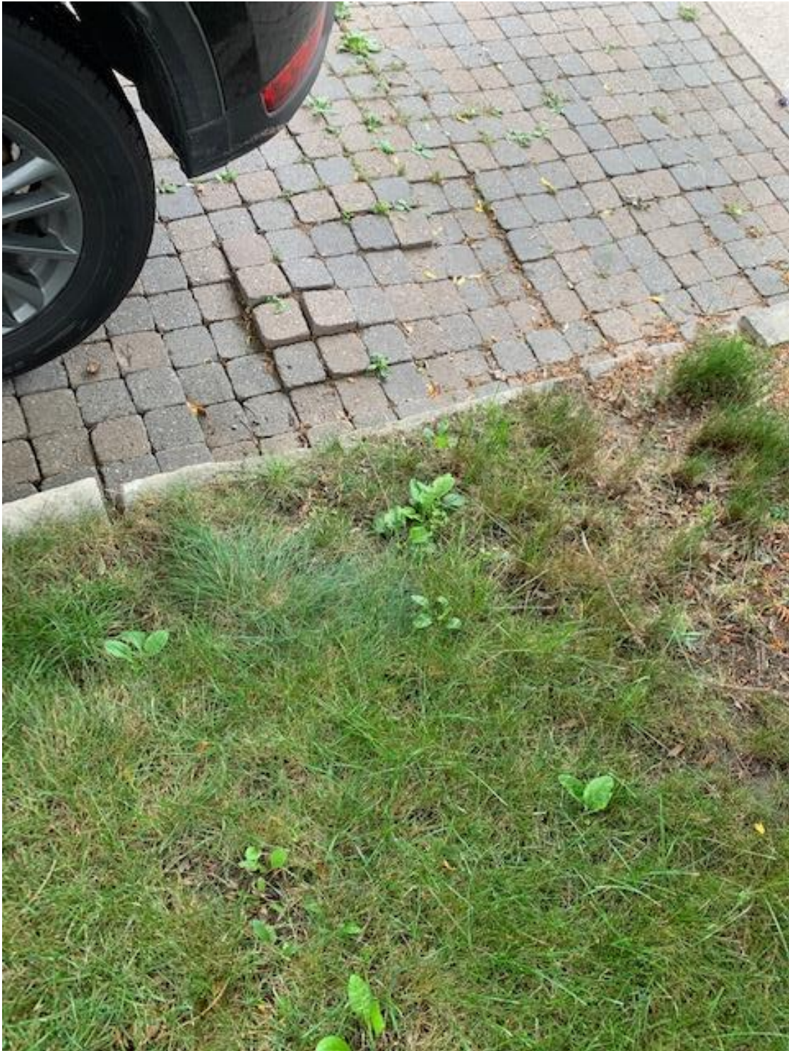
Attachment 2 – Figure 2: Staff photograph showing lifted driveway patio stones at 343 Runnymede Road; July 13, 2021
