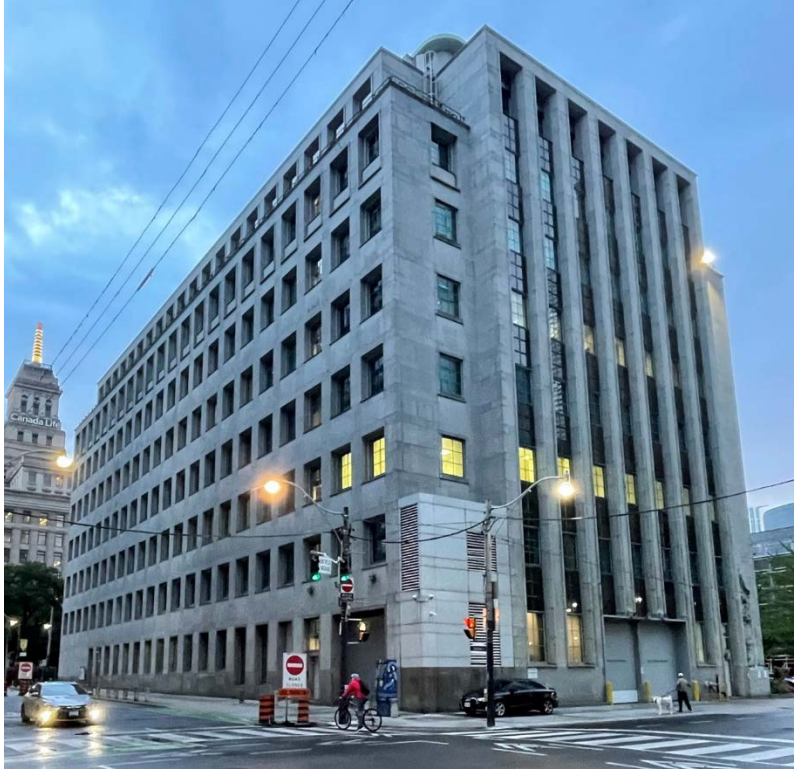
250 University Avenue, south and west façades. Heritage Planning, 2021.
