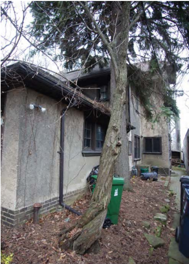
View of North (side) elevation.
