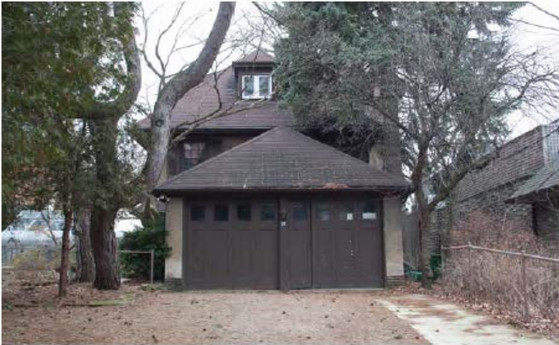
Photograph of the east elevation (front) of the existing house as seen from the street
