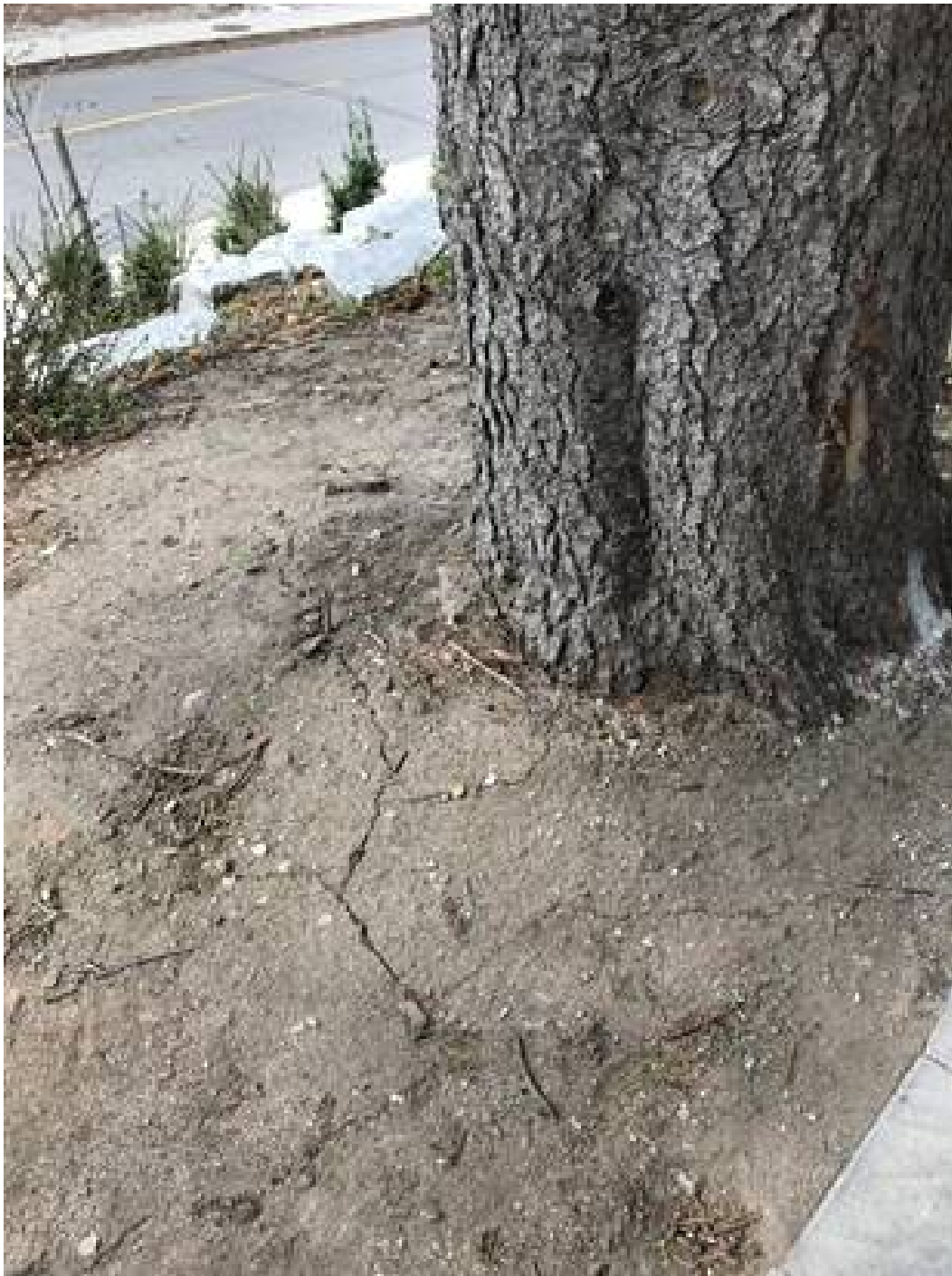
Attachment 2 – Figure 2: Homeowner photograph showing soil cracks at the base of the white spruce tree at 351 Kennedy Avenue; 2018
