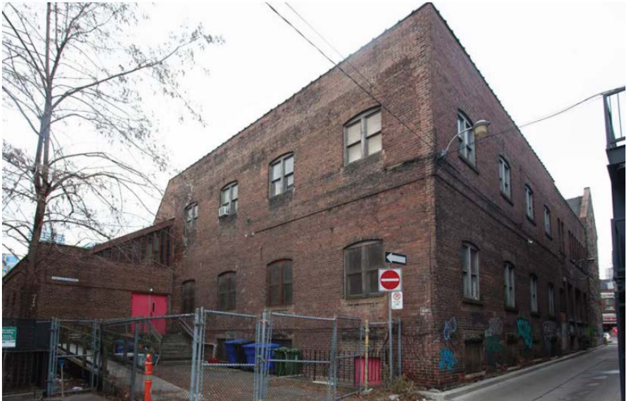
View of the east and south elevations of the Sunday school (Source: ERA Architects)
