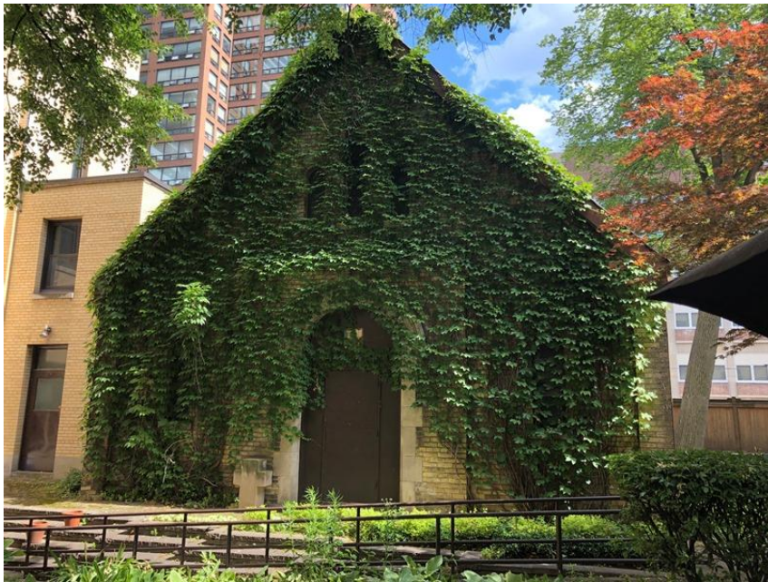
5. Newman Chapel, principal, north elevation facing the west courtyard (Heritage Planning, 2020)
