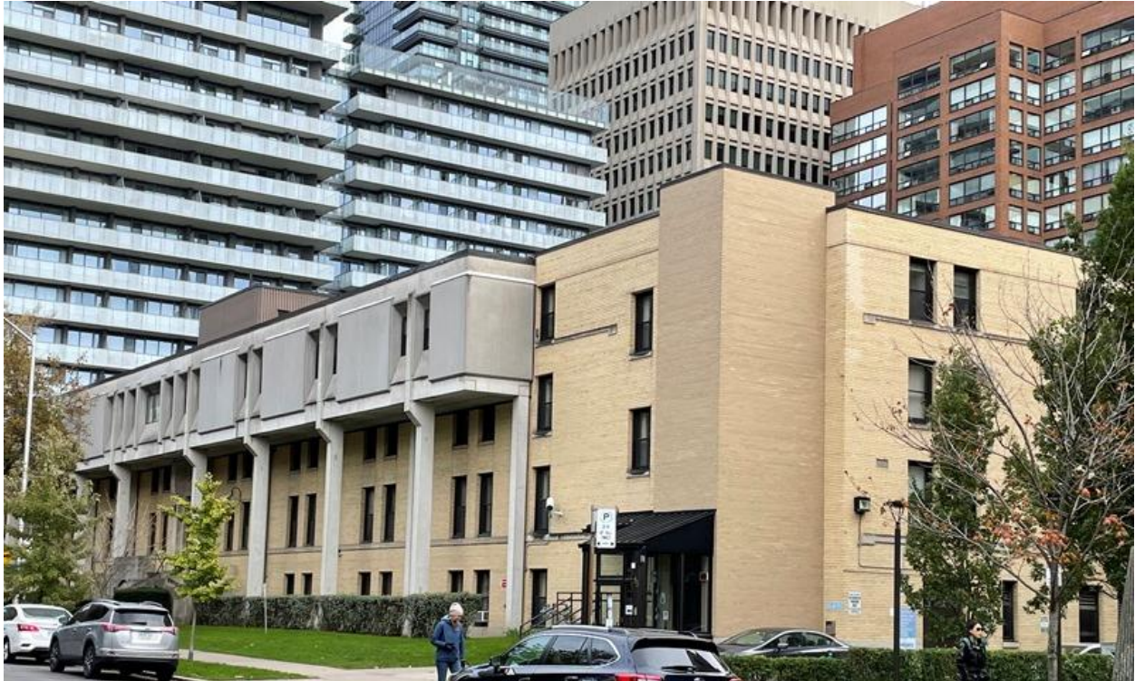
3. St. Basil's Seminary, principal (north) façade and side (west) façade with later stair tower and glazed entrance at the corner. (Heritage Planning, 2021)
