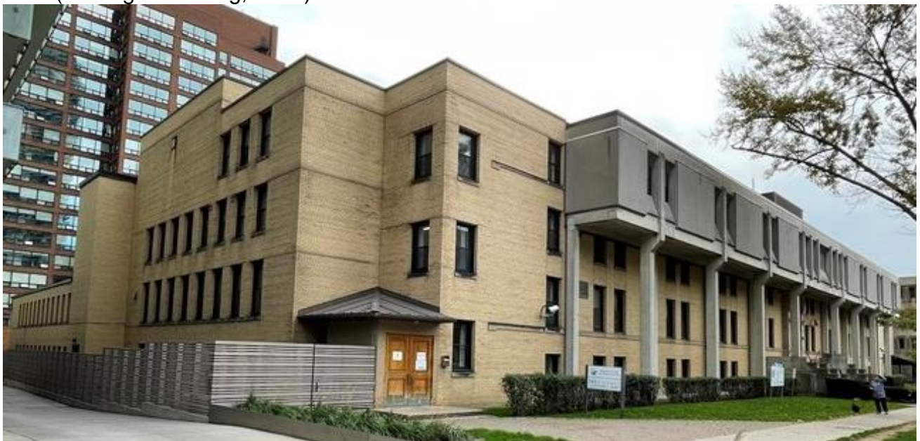
2. St. Basil's Seminary, side (east) and principal (north) facades with later additions including the two-storey extension (far left), 4th floor extension on the north elevation and the new single storey entrance. (Heritage Planning, 2021)
