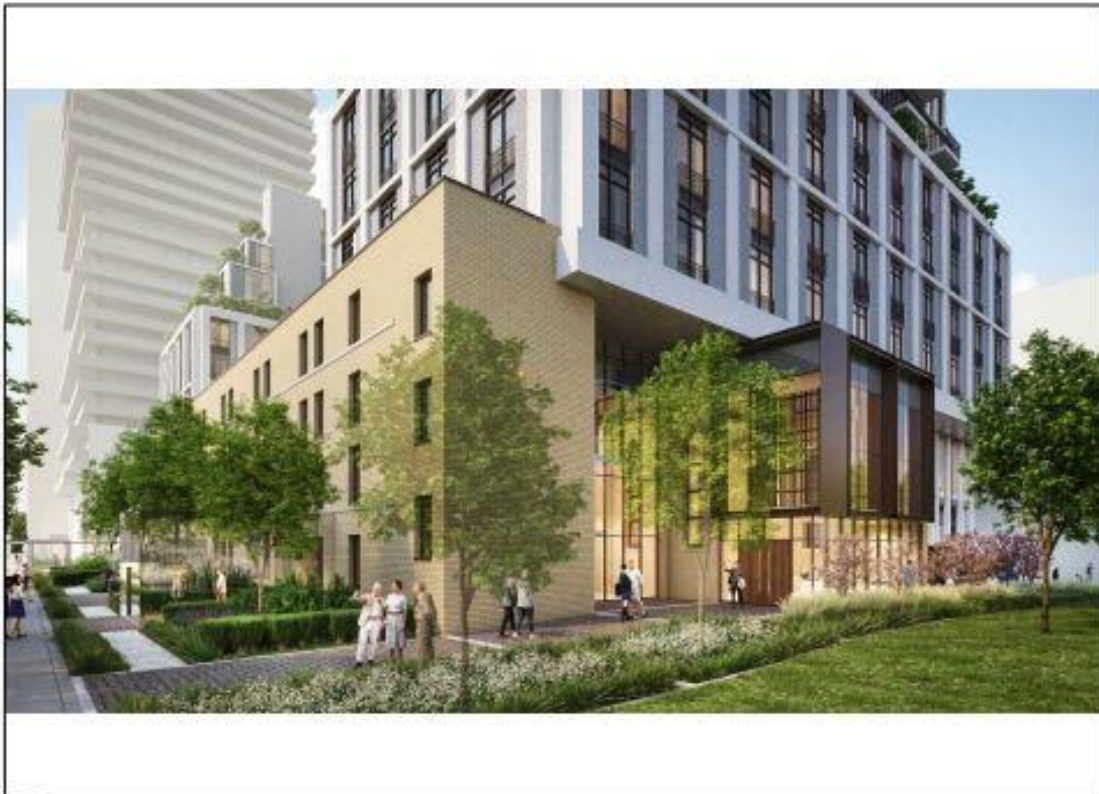
4 NORTH/WEST VIEW FROM ST. JOSEPH STREET
