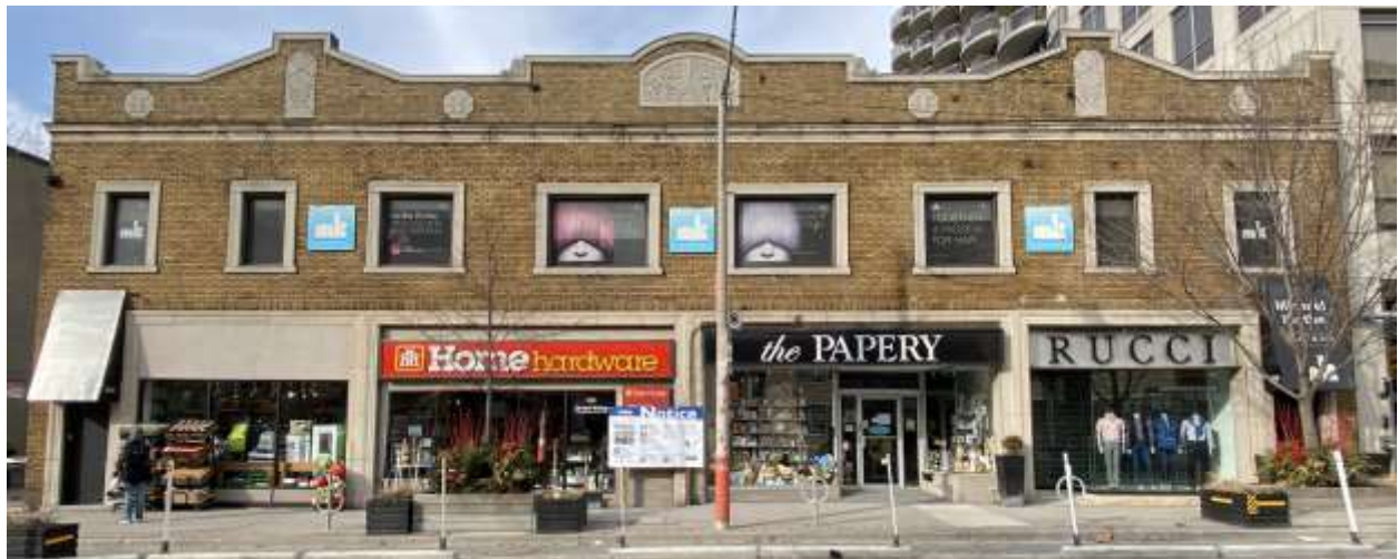
East (primary) elevation of the main street commercial row at 1420 Yonge Street (Heritage Planning, 2022)
