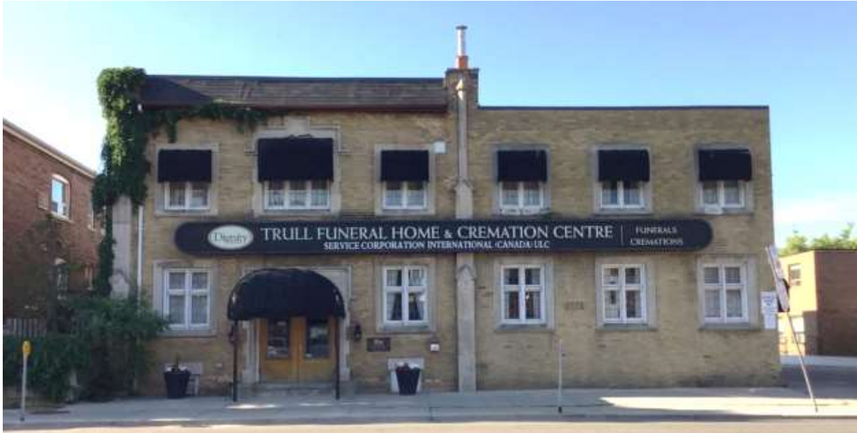
View of the principal (north) elevation of 1111 Danforth Avenue (Heritage Planning, 2020)
