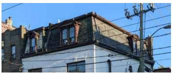
Figure 58: 1402 Queen Street West is a representative example of a property with a mansard roof.
