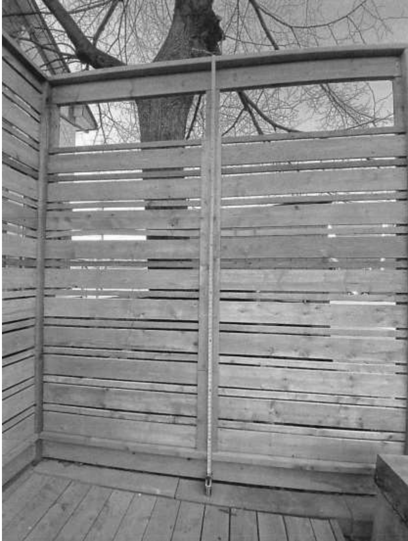
Attachment 3: Measurement of fence
