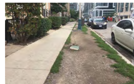
Photo of East Liberty Street boulevard needing repair due to worn-out sod and pedestrian volumes.
