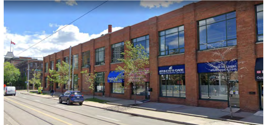
King Street near Dufferin Street: These trees would benefit from the removal of as much paving as possible, to provide larger planting beds for healthier trees.
