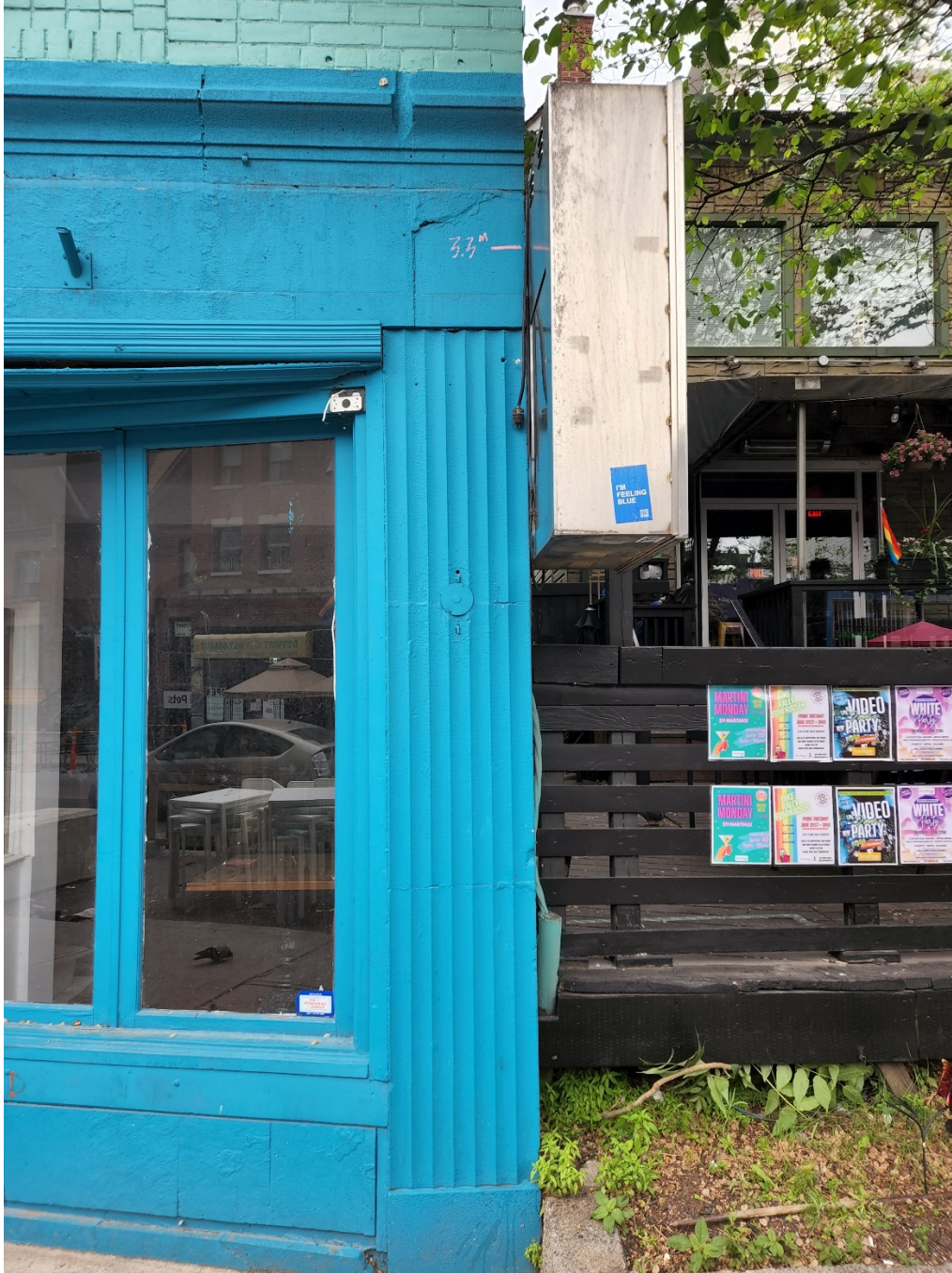
Chalk line approximates the 3.3 meter no building permitted height setback.
