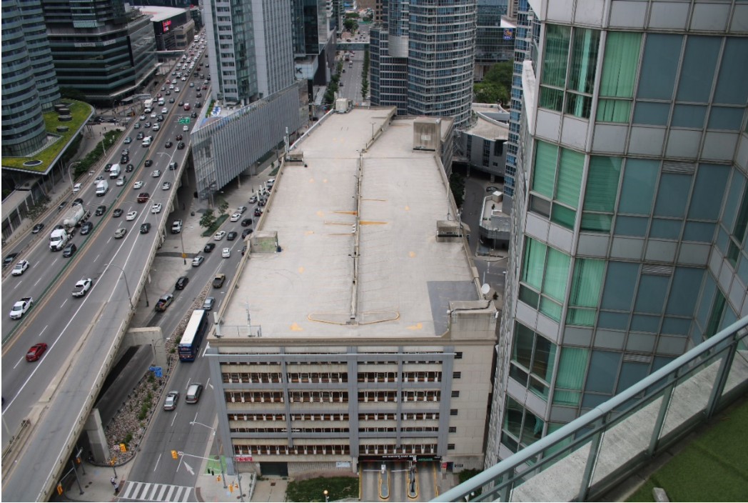
View 1 of parking garage from 228 Queens Quay West, looking east
