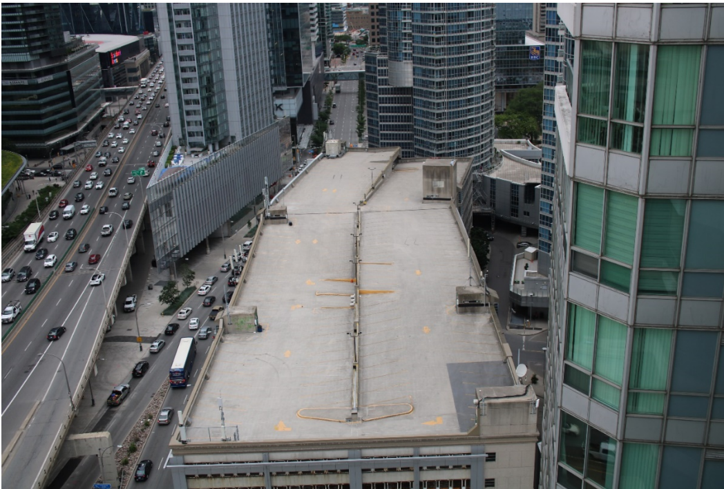
View 2 of parking garage from 228 Queens Quay West looking east
