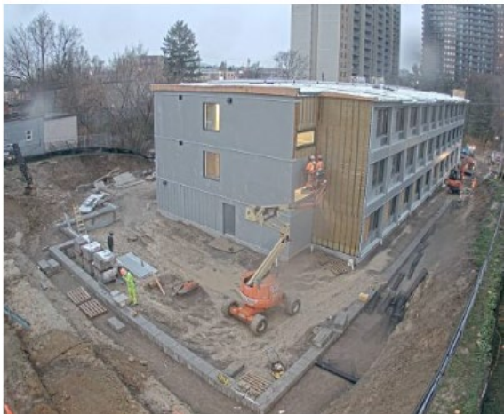
Construction at 11 Macey Avenue
