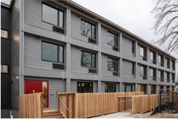
Completed 321 Dovercourt Road
