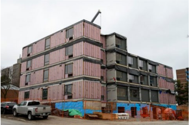
Construction at 39 Dundalk Drive
