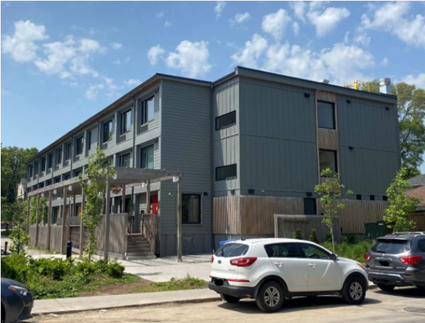
Completed 11 Macey Avenue
