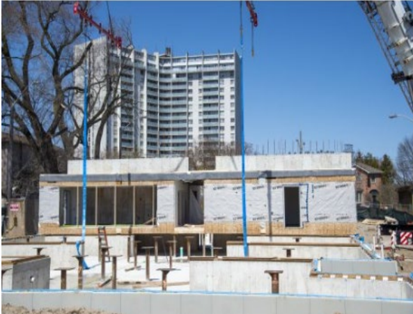
Construction at 540 Cedarvale Avenue
