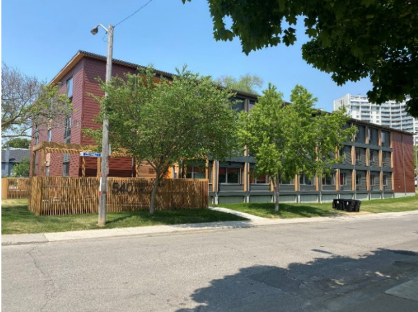
Completed 540 Cedarvale Avenue
