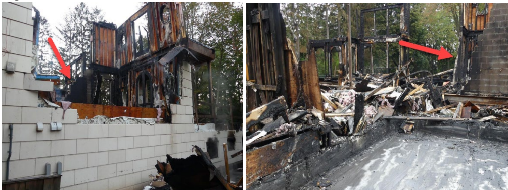
Figure 2: Firewall remains (as shown with red arrows)
