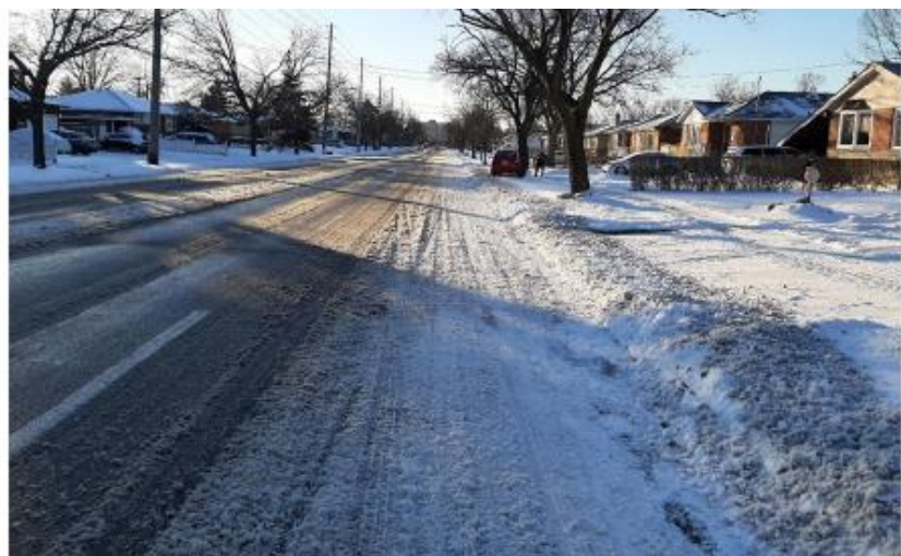
Figure 3: Example of Centre Bare Pavement Conditions
