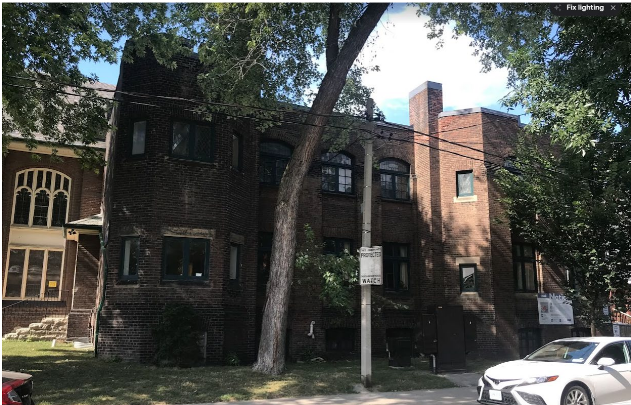
Image 19. The 1907 Sunday School wing plus 1914 eastern addition at right (Heritage Planning, 2022)
