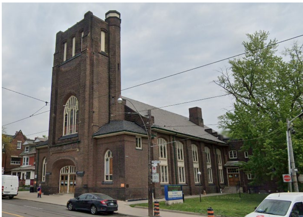
Current image showing the principal (west) and south elevations of St. John's Presbyterian Church.
