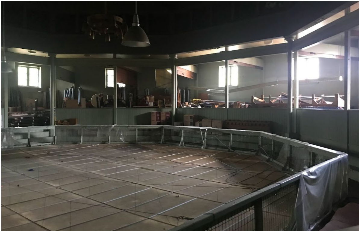
Image 40. Current interior of the semi-circular apse space (gallery level) at the east end of the building (Heritage Planning, 2022)
