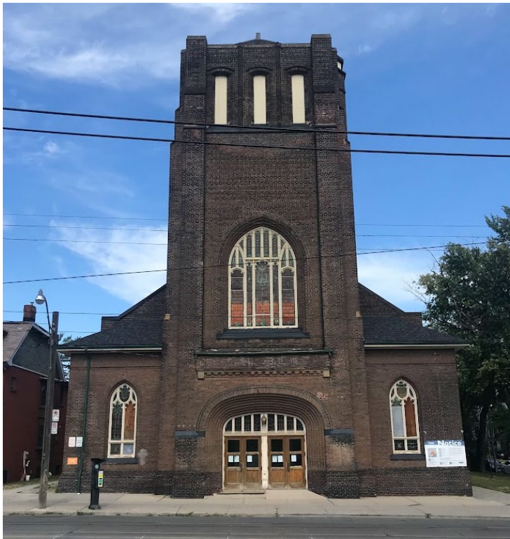
Image 13. Principal (west) elevation of the church with its centred tower and flanking transepts (Heritage Planning, 2022)
