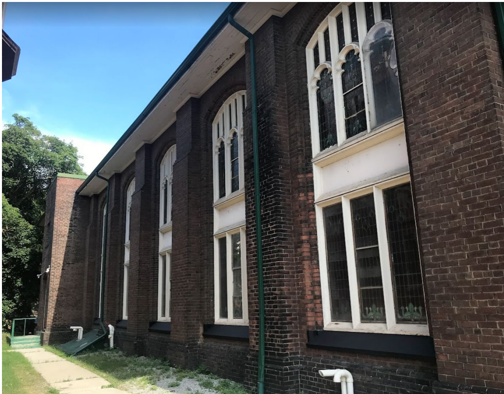
Image 17. Detail of the north elevation (Heritage Planning, 2022)
