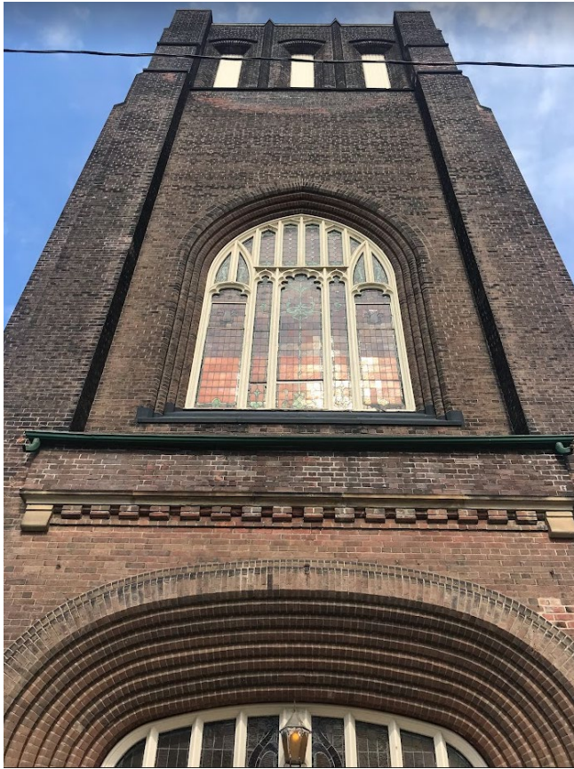
Image 14. Detail of the tower on the principal (west) elevation, showing the Neo-Gothic openings (Heritage Planning, 2022)
