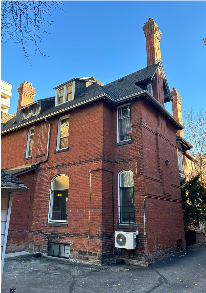
Figure 15: North (rear) and west elevations of 94 Isabella Street (Heritage Planning, 2022).
