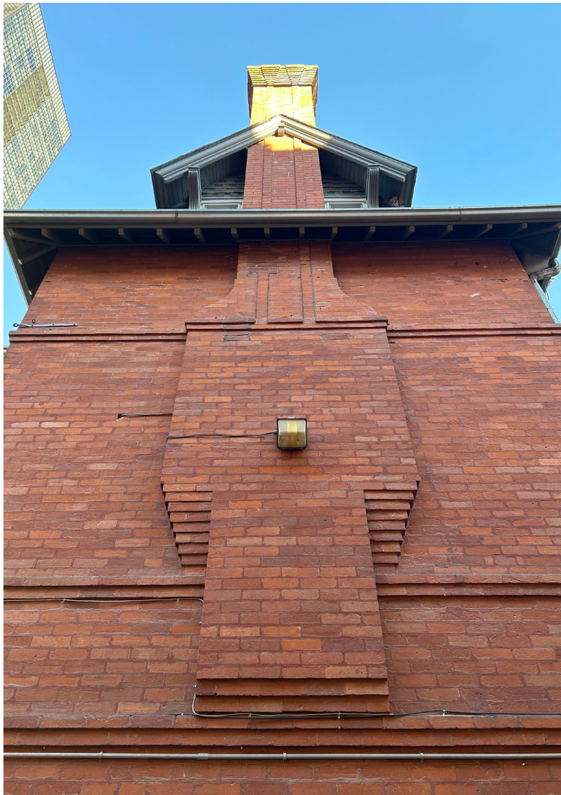
Figure 14: Corbelled brick chimney on west elevation of 94 Isabella Street (Heritage Planning, 2022).
