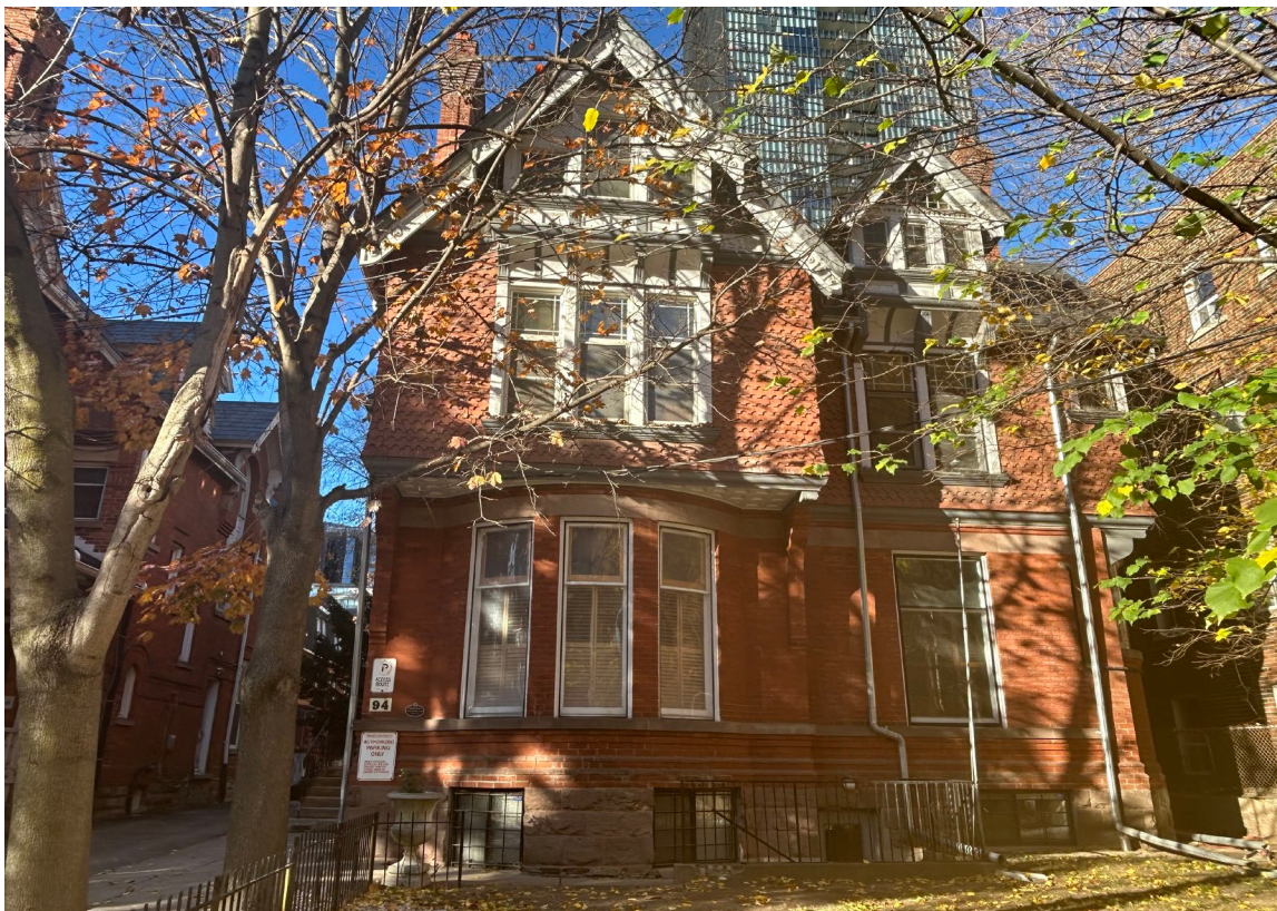
Figure 10: South elevation of 94 Isabella Street (Heritage Planning 2022).
