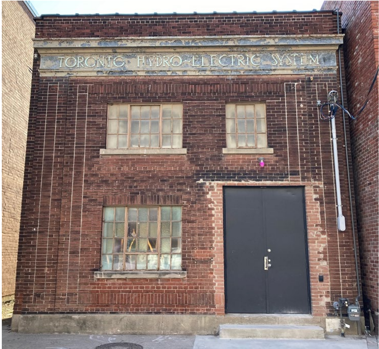
18 Portland Street. Principal (east) elevation. Heritage Planning, 2022.
