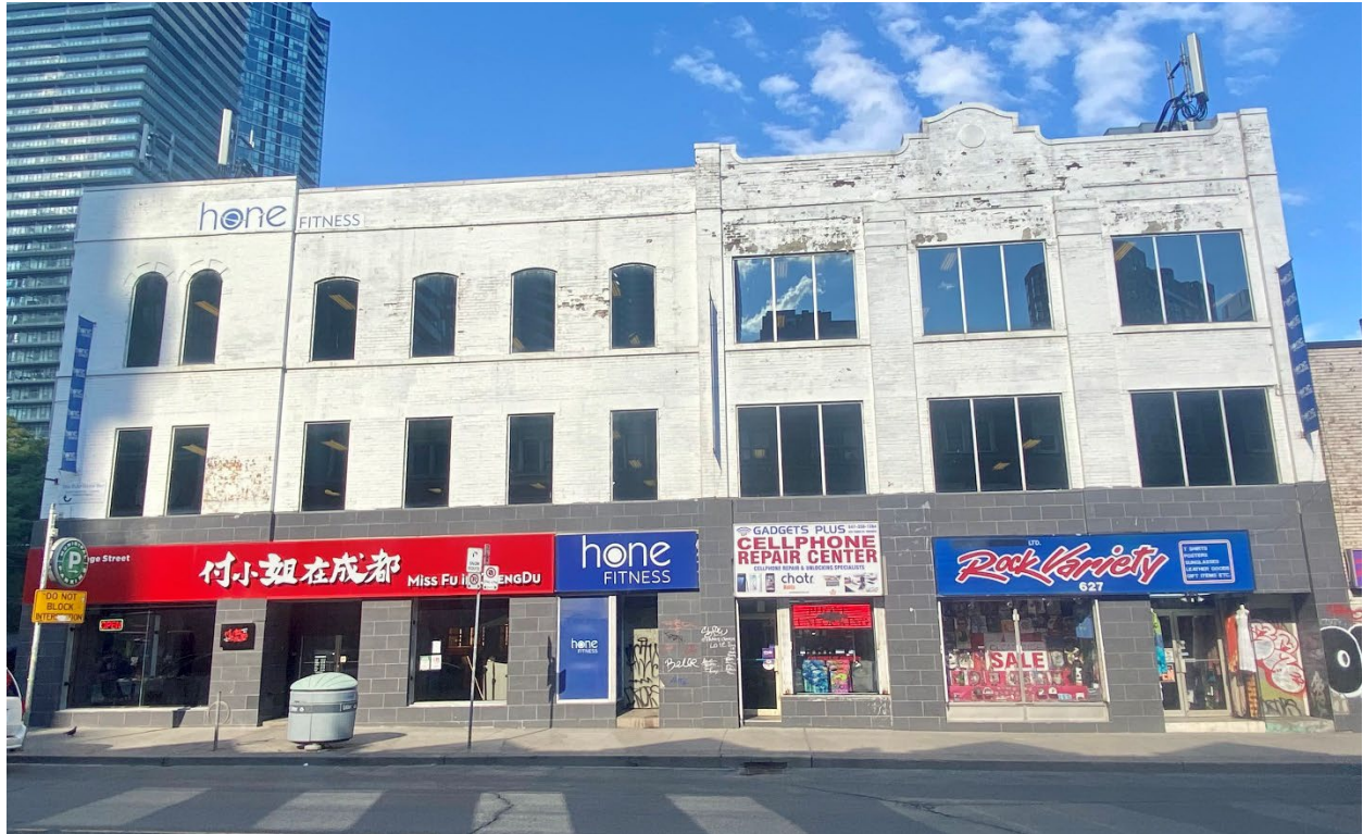
West elevation of 625 Yonge Street, facing Yonge; northern building (631-637 Yonge Street/1-5 Isabella Street) at left, and southern building (625-629 Yonge Street) at right (Heritage Planning, 2022).
