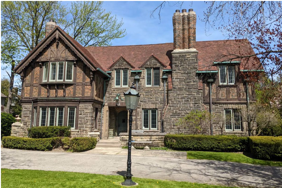
Image 18. Current photo showing the west elevation (ERA, 2022)
