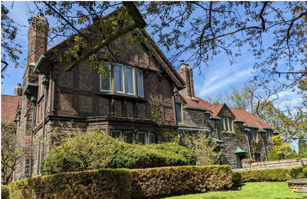
Image 19. Current photo showing the west and partial south elevations (ERA, 2022)
