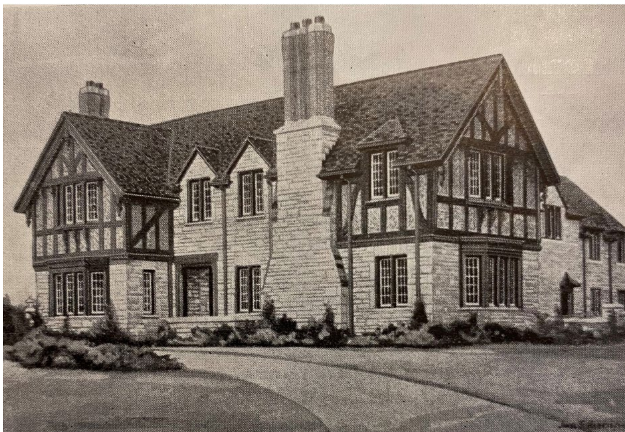
Image of the Dorothy (McLaughlin) Tait House at 63 Old Forest Hill Road as it appeared in Canadian Homes and Gardens , XIII, Jan/Feb 1936, page 39, and showing the principal (west) and south elevations.
