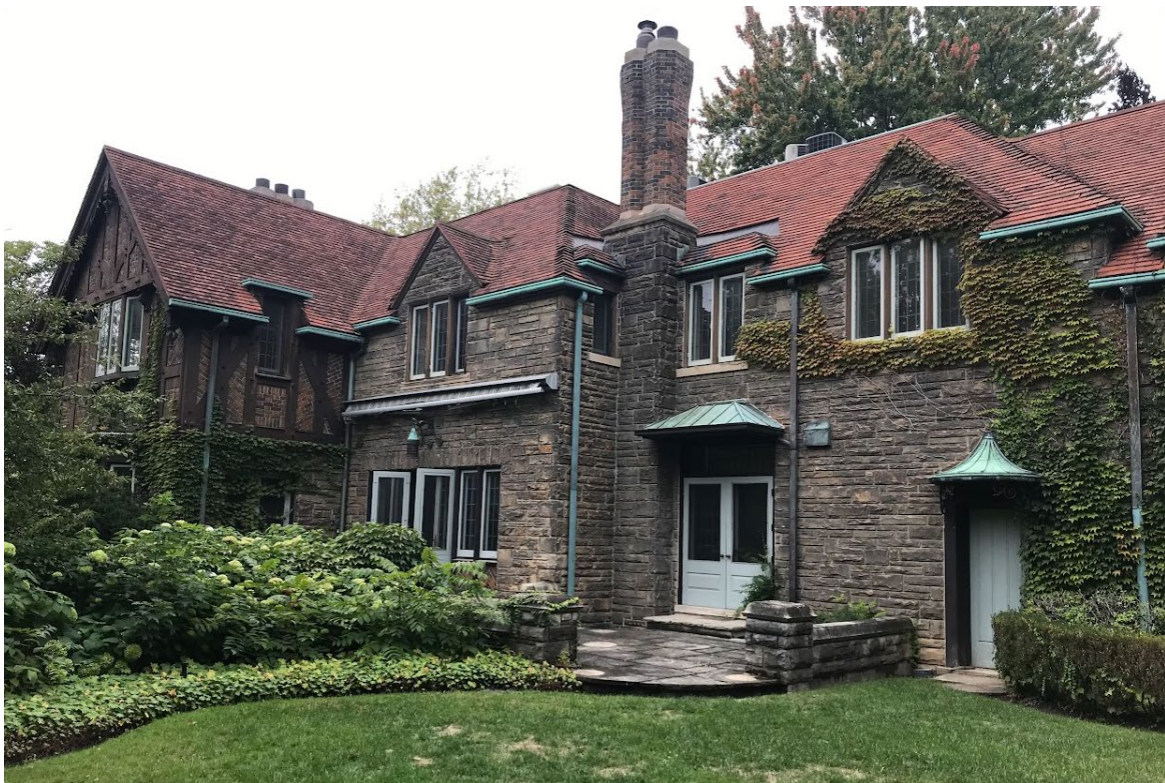
Image 28. Detail of the south elevation, looking northwest and showing the 1990s garden terrace extension and new double door opening with hipped copper roof at centre (Heritage Planning, 2022)
