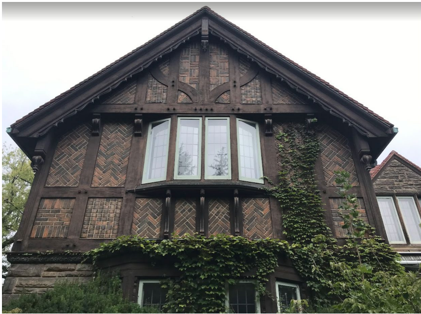
Image 23. The roof gable on the west elevation showing the half-timbering, wood detailing and mirrored brick infill patterns (Heritage Planning, 2022)
