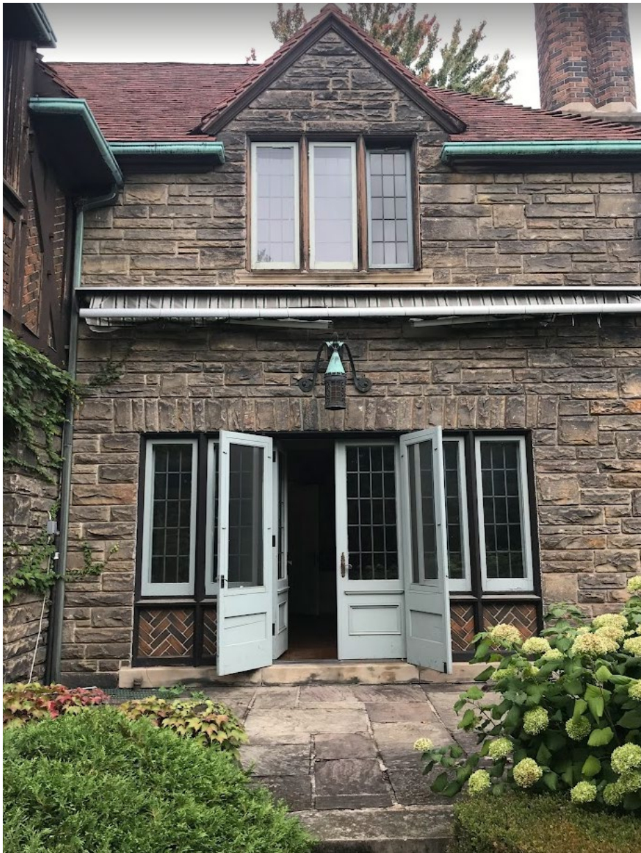
Image 25. The original French doors on the south elevation and flagstone garden terrace, looking north (Heritage Planning, 2022)
