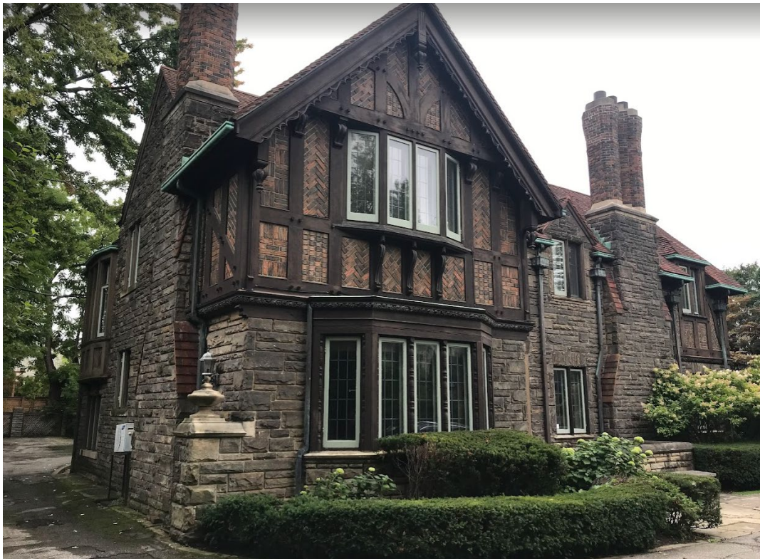
Image 21. Current photo showing the west and partial north elevations (Heritage Planning, 2022)
