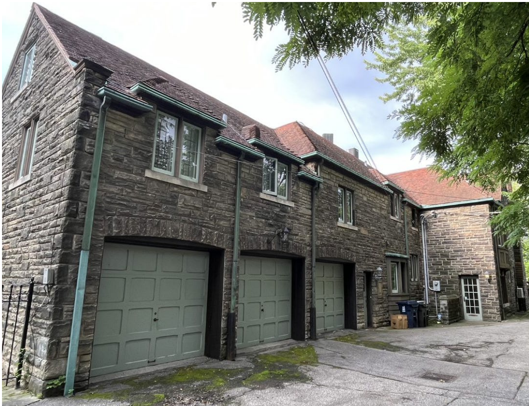
Image 22. Current photo showing the three-car integrated garage (Heritage Planning, 2022)
