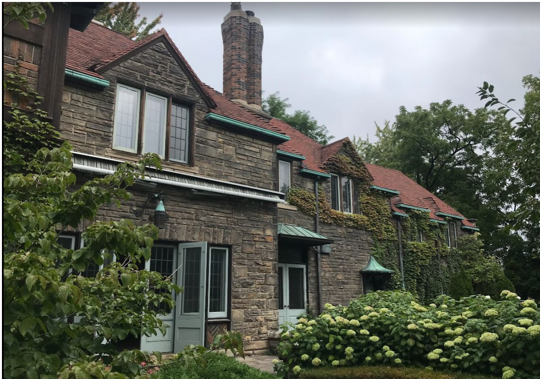
Image 27. Detail of the south elevation, looking northeast (Heritage Planning, 2022)
