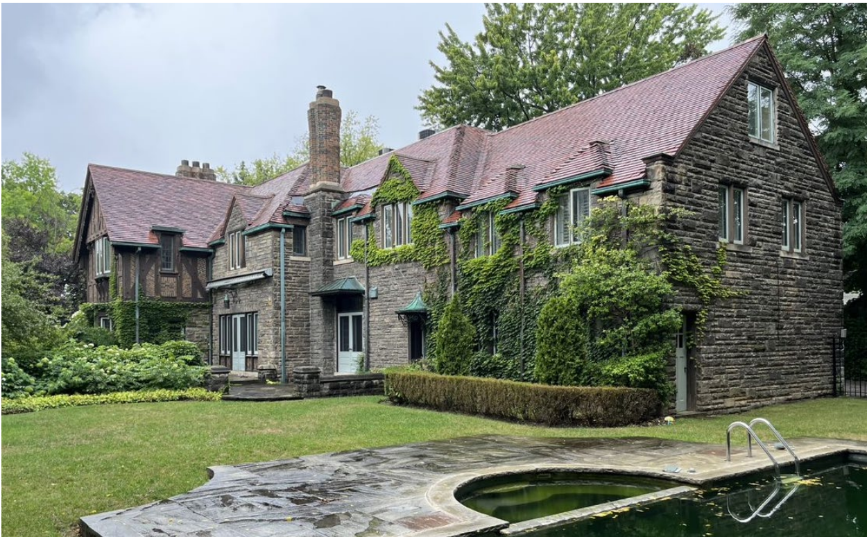
Image 20. Current photo showing the south and east elevations (ERA, 2022)
