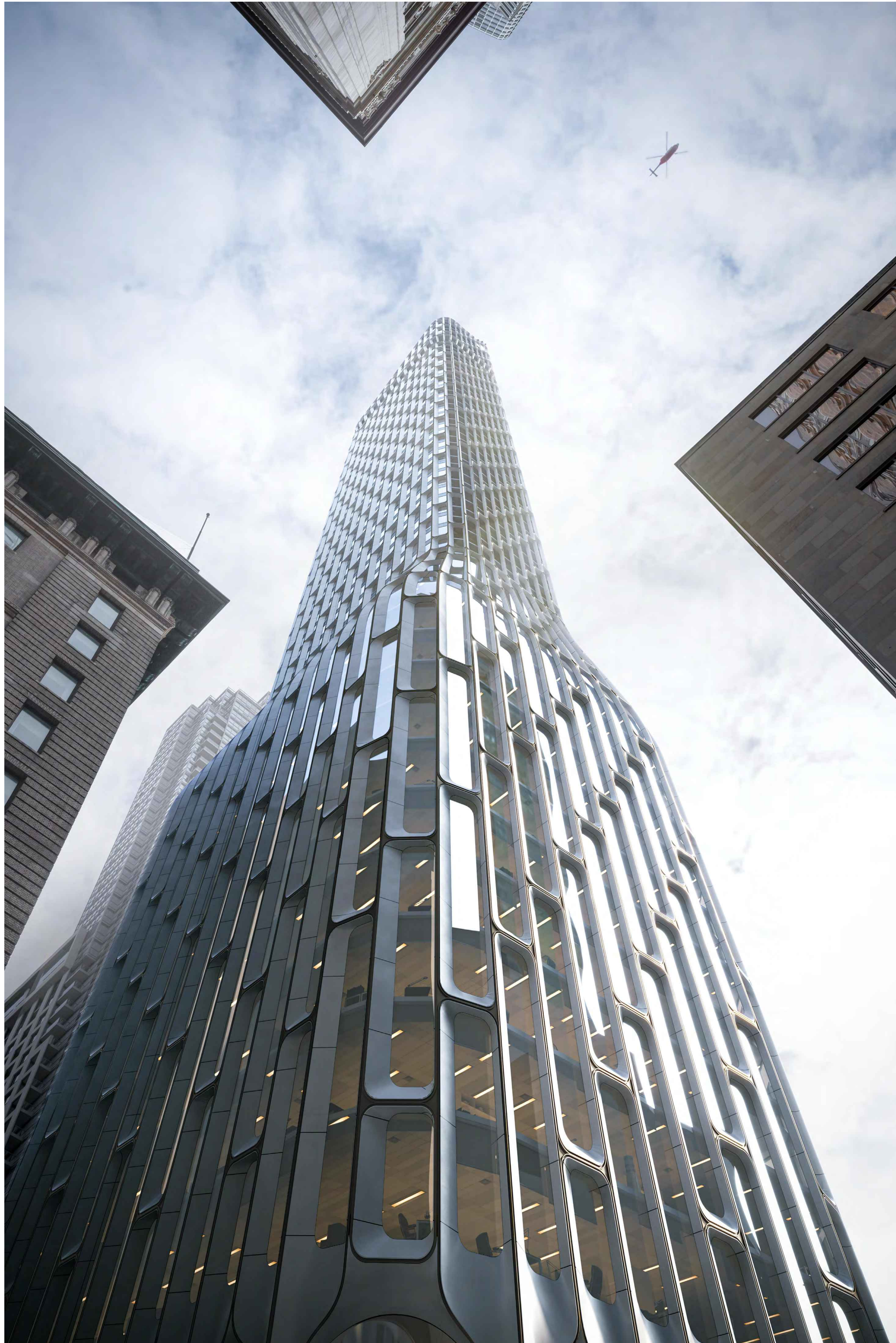
1 A471.S - View of Tower from Yonge Street & Colborne Street
