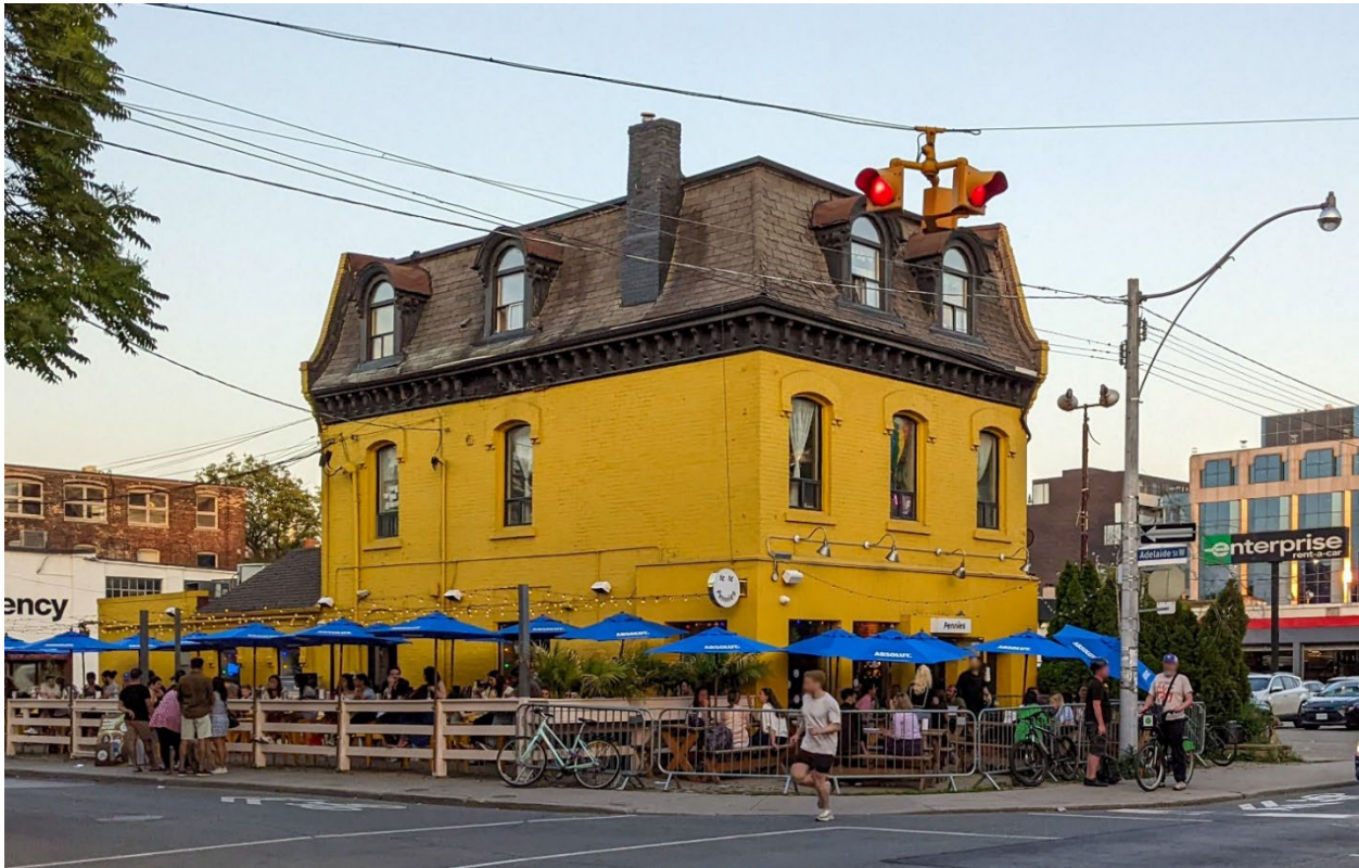
View of the property at 127 Strachan Avenue looking southeast (Heritage Planning, 2022)
