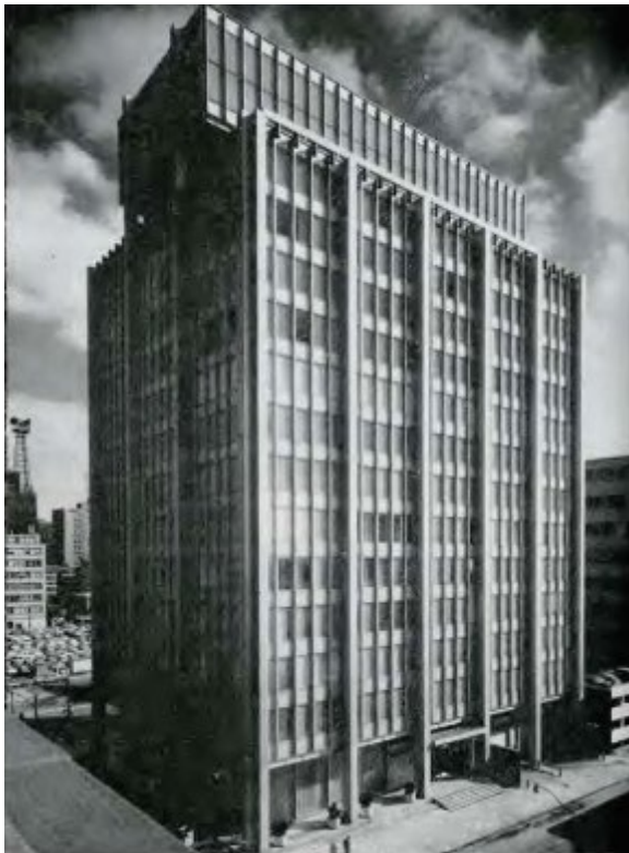
Image 22. 1961 image of the property looking southeast from Simcoe Street and Richmond Street West (RAIC, 1961).
