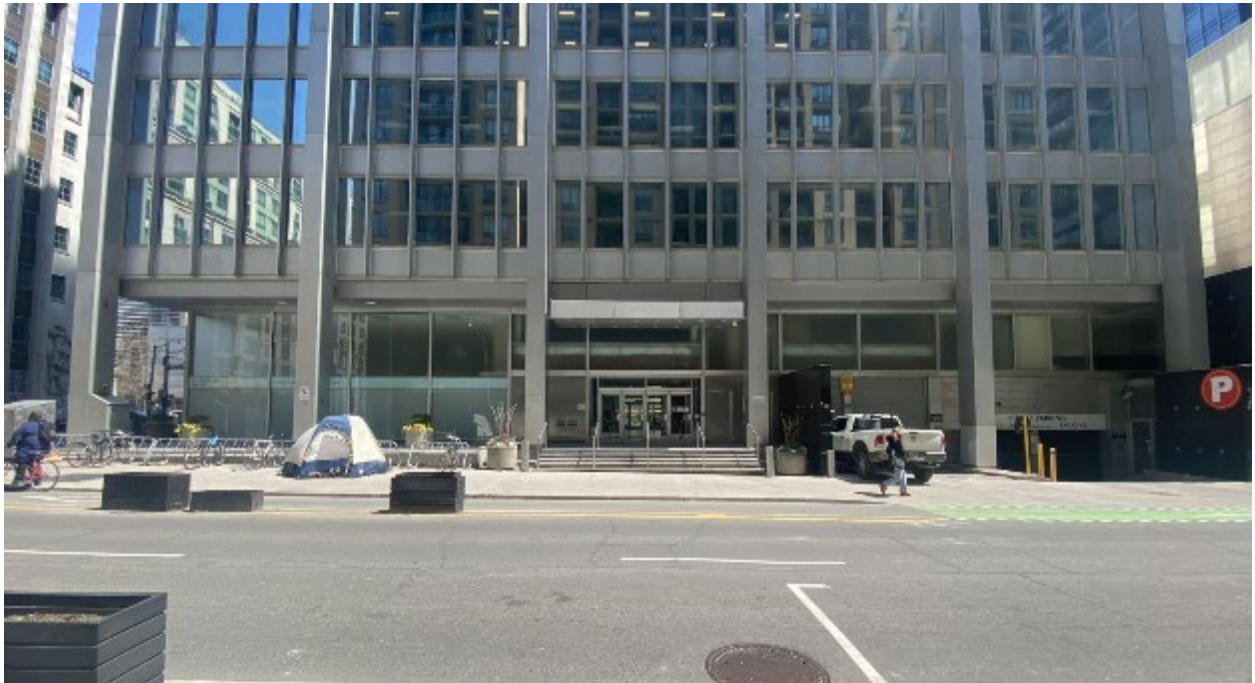
Image 39. Current photo of the west ground floor and mezzanine level set back from the perimeter columns (ERA, 2022)
