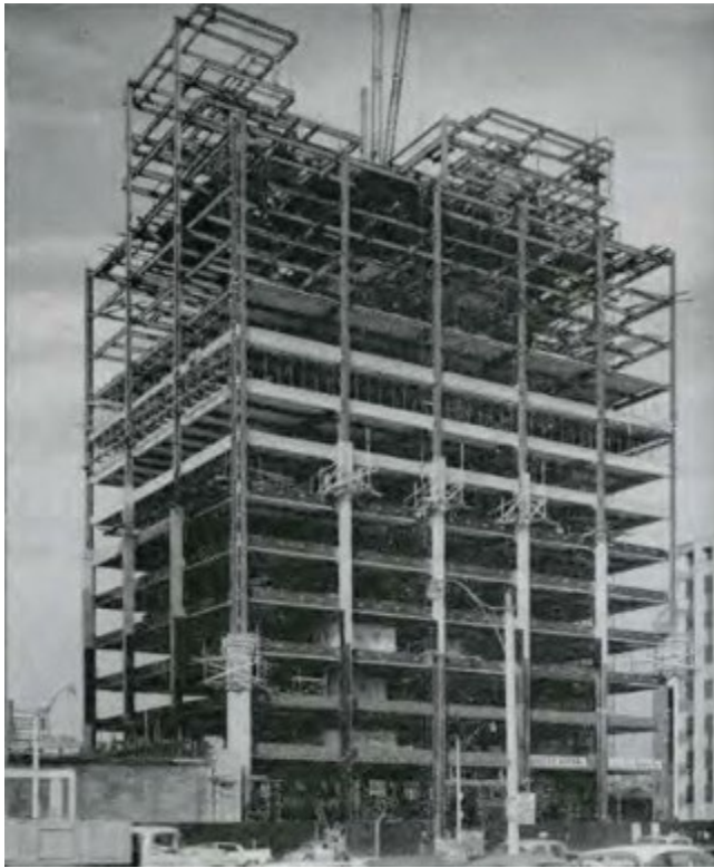
Image 21. 1958-1960 image of superstructure under construction (RAIC, 1961).
