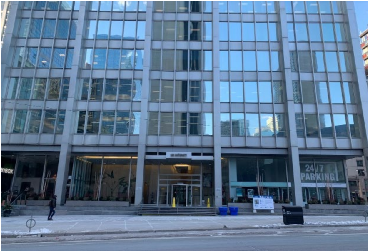
Image 38. Current photo of the east ground floor and mezzanine level set back from the perimeter columns (Heritage Planning, 2023)
