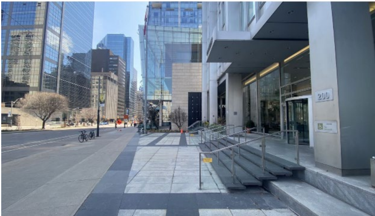
Image 36. Current photo looking south along University Avenue and showing the granite public plaza and main entrance with aluminum-clad canopy and floating granite steps in front of the main entrance of the Sun Life Building (ERA, 2022)
