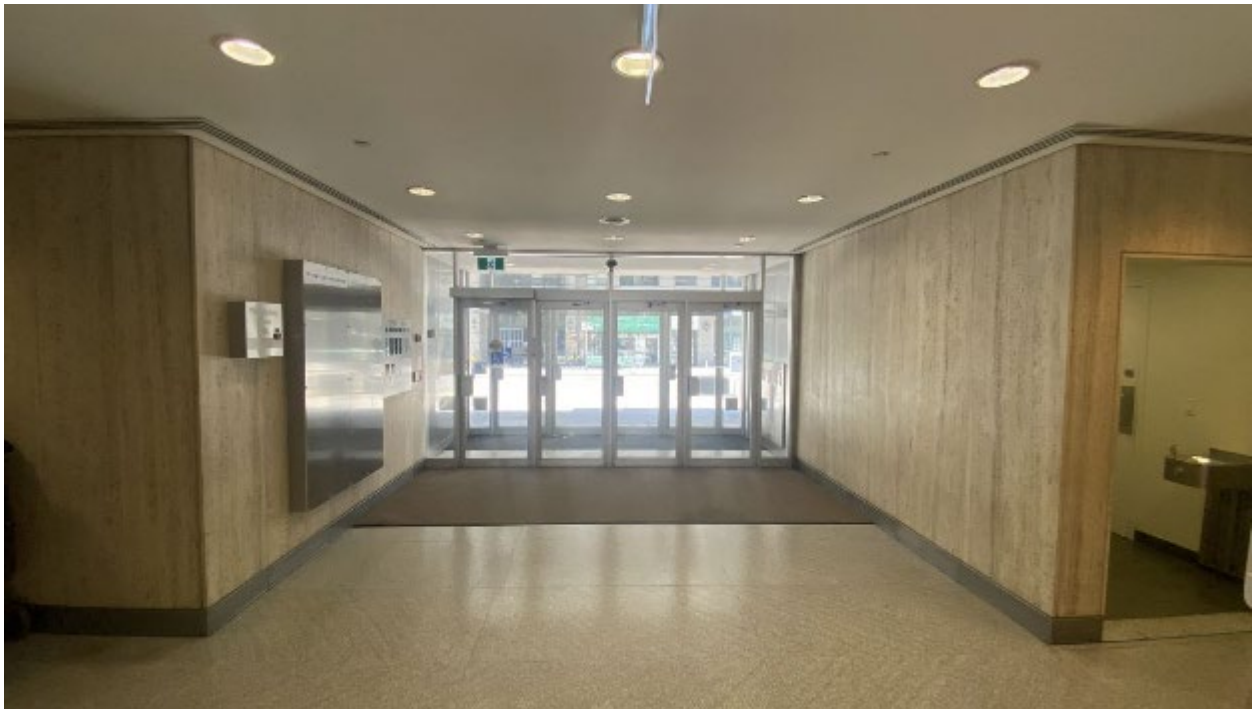
Image 44. Current photo looking west across the elevator lobby to the Simcoe Street entrance and showing the travertine wall panelling, granite floors and stainless steel elevator doors and surrounds. (ERA, 2022)
