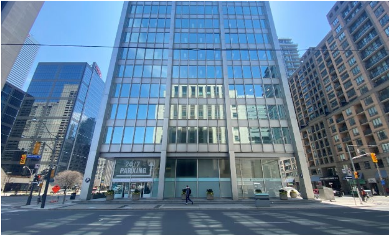
Image 31. Current photo of the north elevation (ERA, 2022)
