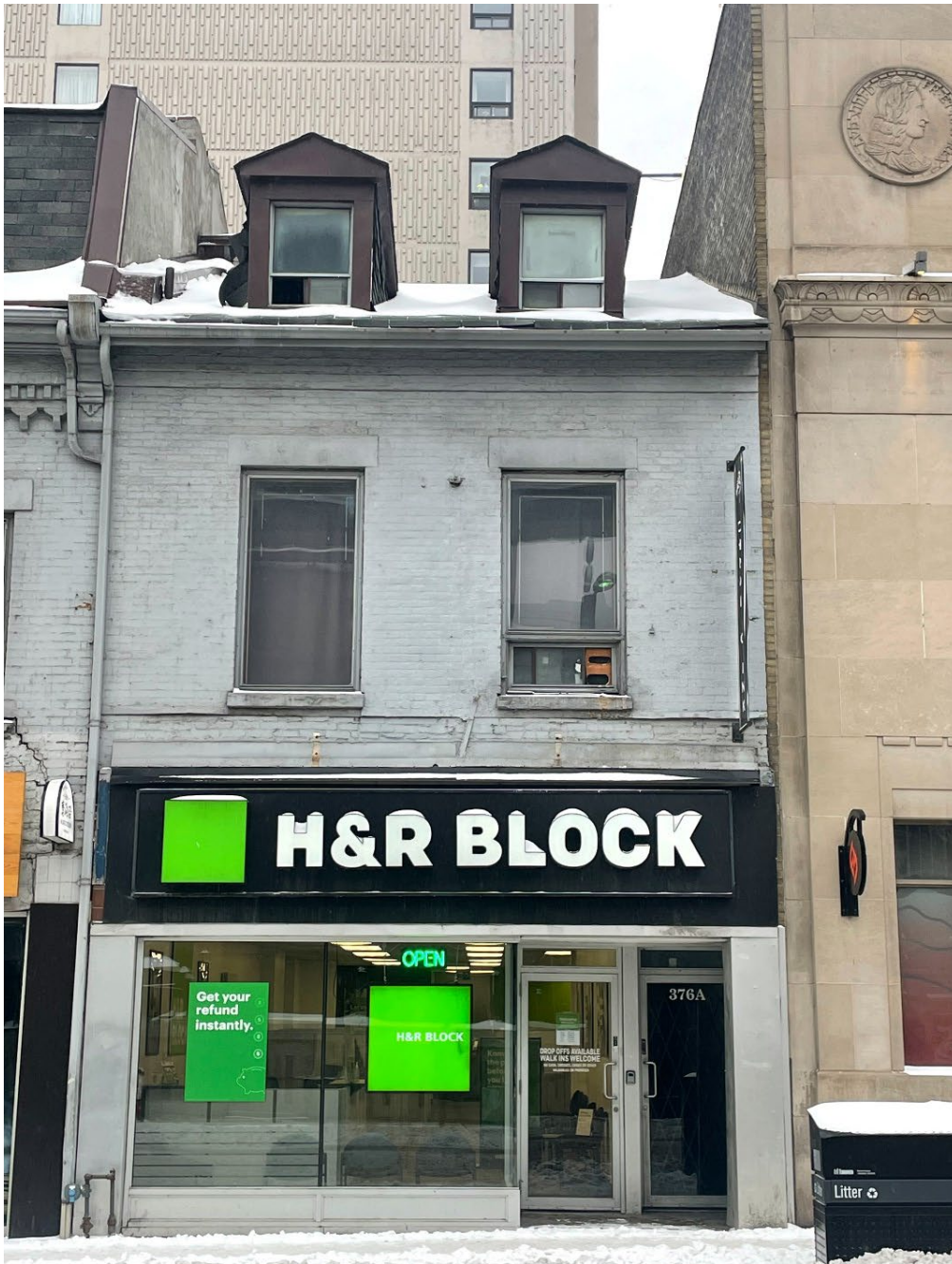
Figure 10: East elevation of 376 Yonge Street, 2023 (Heritage Planning)
