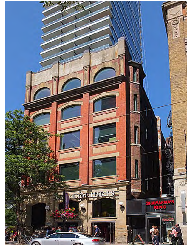
106. 220 King W from the SE. Note the missing cornice at the area of cement parging at the 5th floor, a projecting cornice will be restored. Recessed in the gap between 220 and 218 to the right there will be infill with a glass south wall located behind the projecting oriel window. The current street related infill will be removed. PGA
