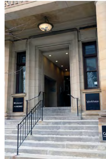
53. Stairs (11 steps) leading up to the main doorway opening within the portico off King W. Note the recessed entrance doors within building. PGA
