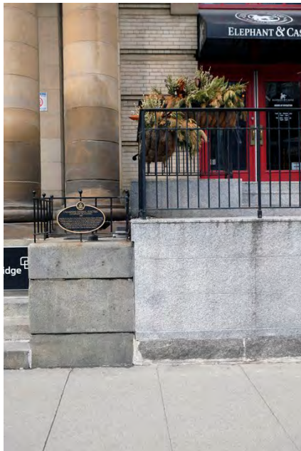
54. Detail of portico pedestal, left, at concrete stair addition to a new commercial entrance, right. PGA
