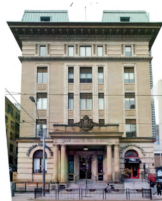
49. South elevation 212 King St W. PGA
