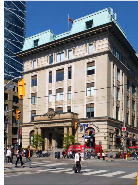
94. View of 212 King from SE corner. PGA
