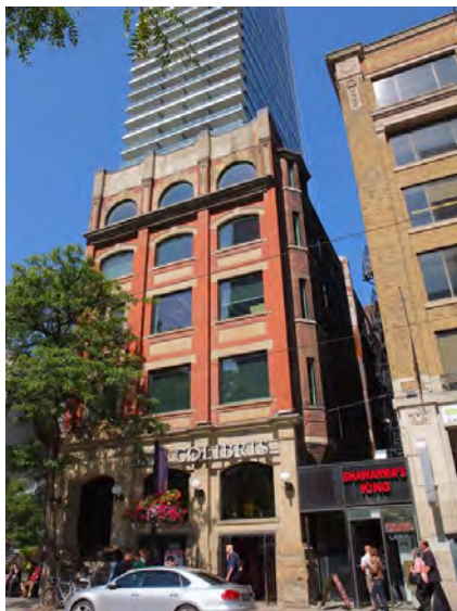
45. 220 King W south elevation on King W. PGA
