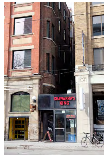
69. 220 King W. view into the gap between 218 King W. The shallow oriel window is visible. A new glazed infill wall is proposed between these buildings set back beyond the oriel window, the current infill will be removed. PGA
