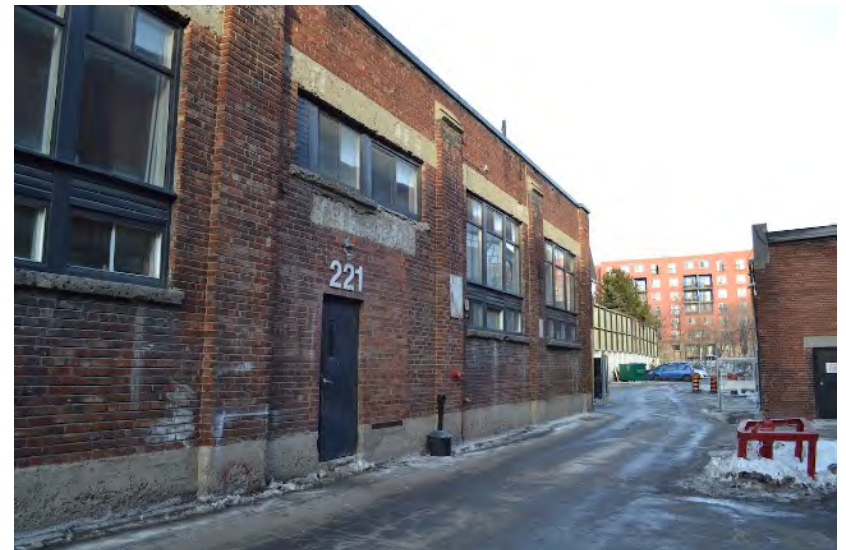
Figure 4 - View of the south facade of Building C (east).
