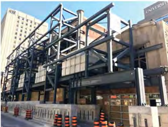
External two and three storey bridged over hydro vault
