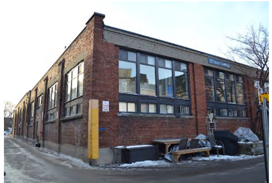
Corner of the south (left) and east(right) elevations. Window opening sizes and locations differ, as well as the wall compositions (on the east elevation, the concrete lintels are continuous along the length of the building, whether on the south elevation, lintels are interrupted). Sills on the east elevation are heavily eroded and do not project as much as the sills on the south elevation, resulting in more notable water run-off. In either case, the sills are lacking proper dip cuts/ groves to break the flow of water.
