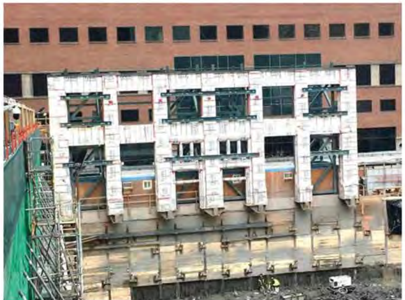
Cantilevered retention, interior needle beams
