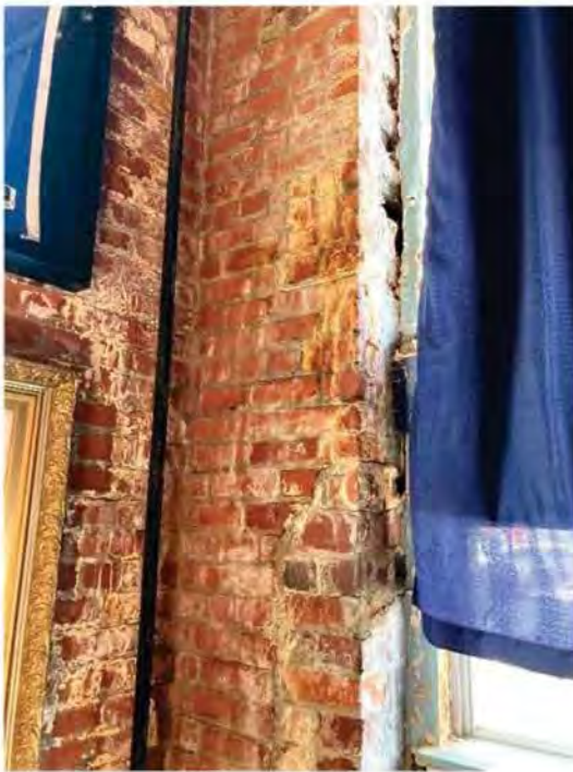
BLDG C WEST – INT SOUTH WEST CORNER 2
