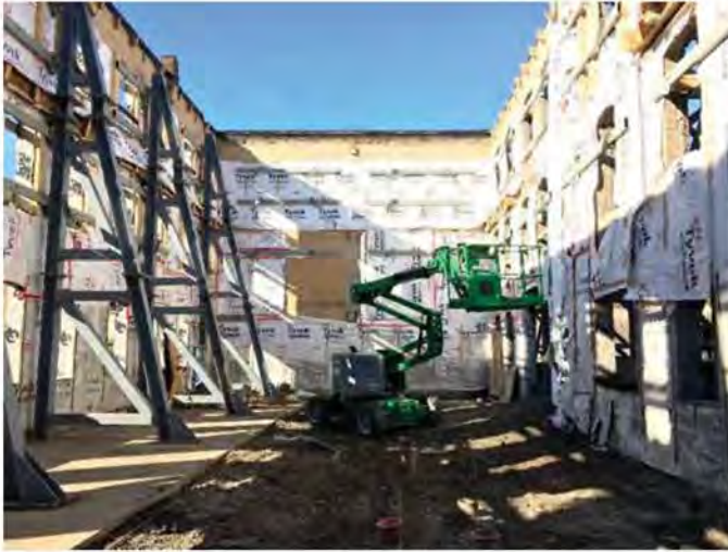
495 King St W – Interior, south elevation
