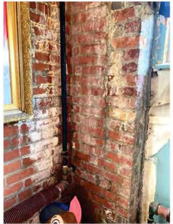
BLDG C WEST – INT SOUTH WEST CORNER 3
