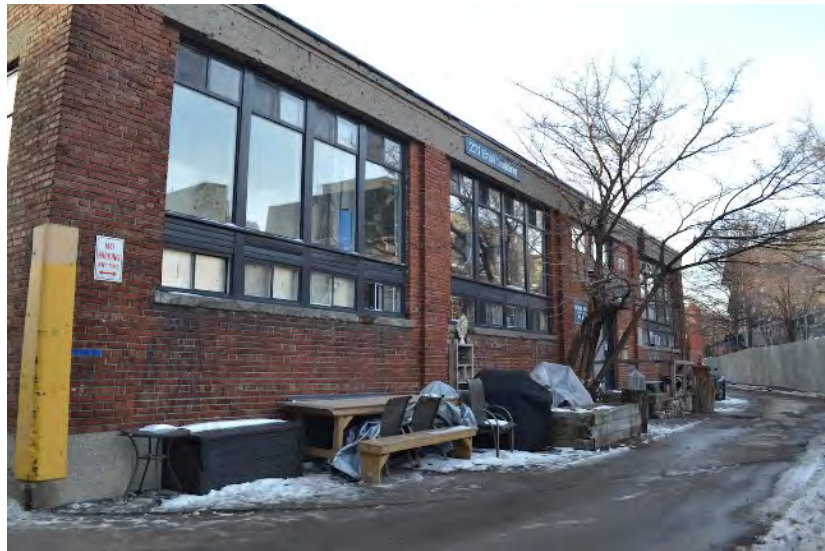
Figure 5 -View of the east facade, Building C (east).
