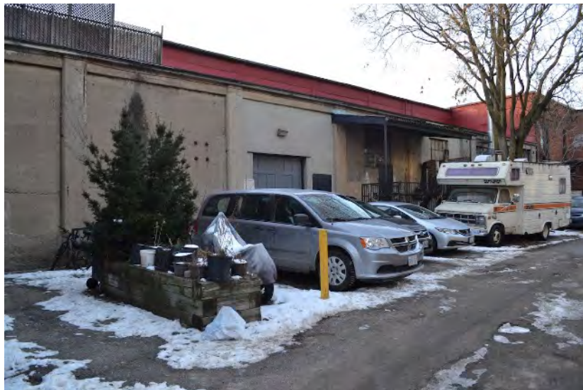
Figure 10 - View of the unnamed lane to the east of the subject site, showing the east facade of Building B (west).
