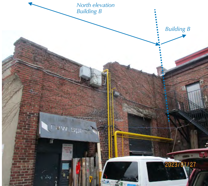
North elevation, showing two original service door openings with new infills and the removed brick pilaster of east elevation now parged (on the left of the photo). Building B is visible at the right of the photo.
