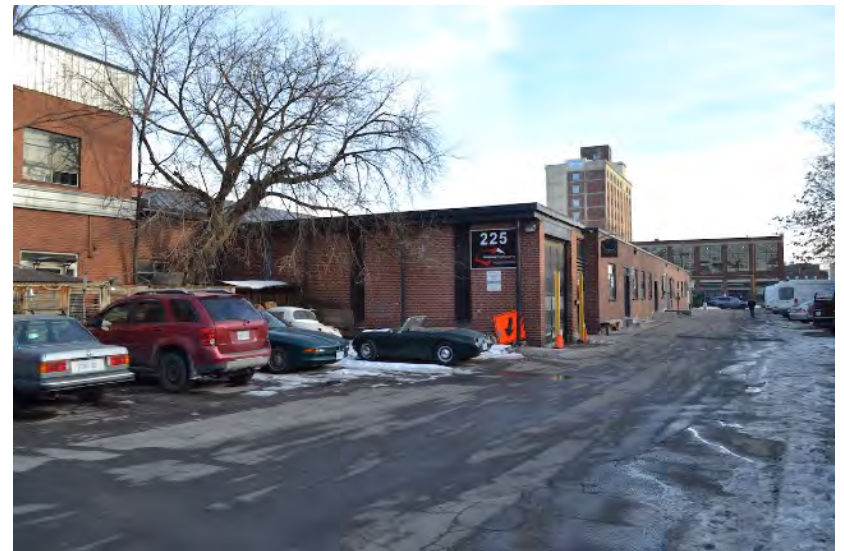
Figure 16 - View of the unnamed lane to the west of subject site, looking south past Building A to Building B (west), showing the former Moloney Electric building and designated property (MOCA) in context.
