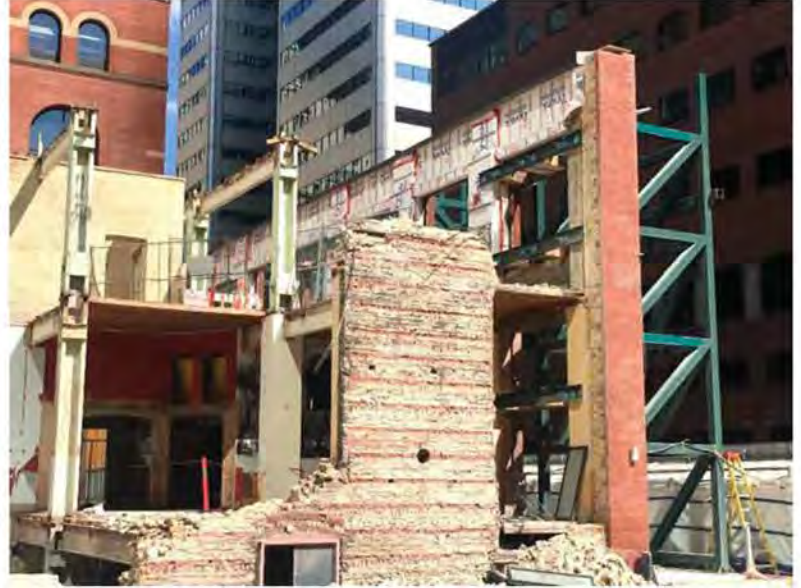
Cantilevered retention on below grade steel support grid
