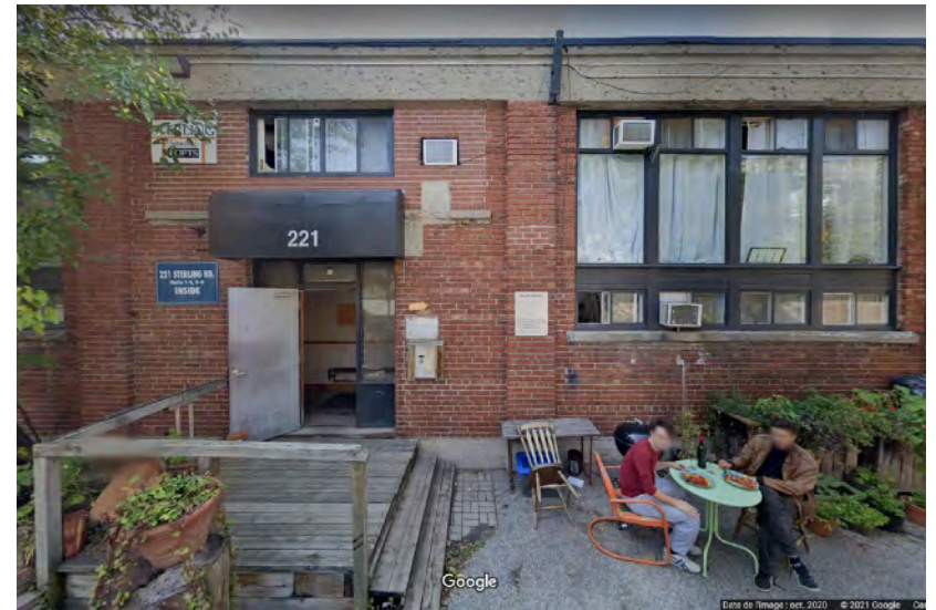
Figure 19 - View of Building C (east), showing the entrance at rear (Google Street View).
