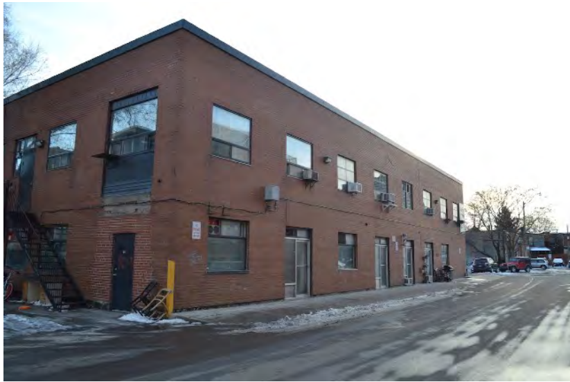
Figure 13 - View of Building A, showing the north facade fronting Merchant Lane.
