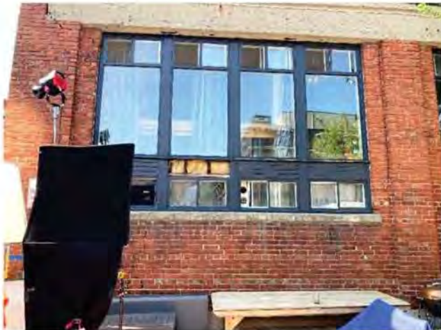
BLDG C EAST – EAST ELEVATION 1
