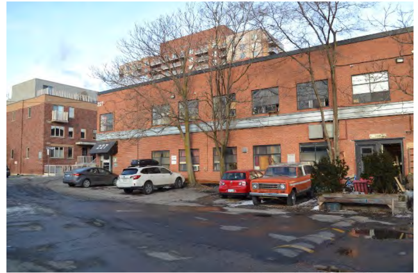
Figure 15 - View of the west facade of Building A.
