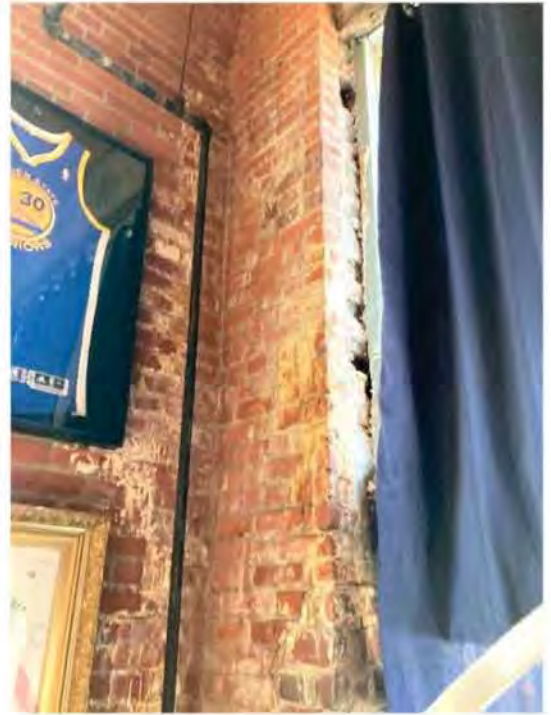
BLDG C WEST – INT SOUTH WEST CORNER 1
