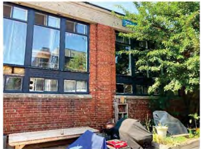
BLDG C EAST – EAST ELEVATION 2
