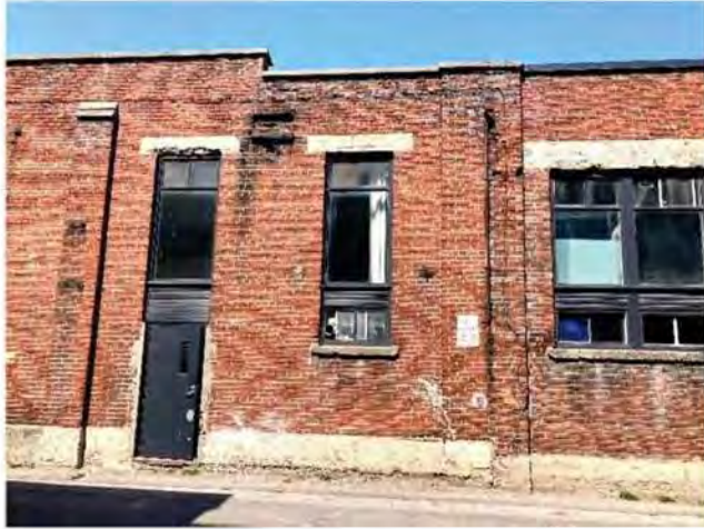
BLDG C WEST – SOUTH ELEVATION
