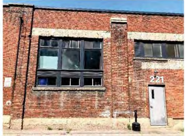
BLDG C EAST – SOUTH ELEVATION
