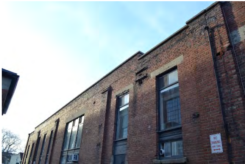
Figure 17 - View of Building C, showing a transition at pilasters between construction phases at the south elevation.
