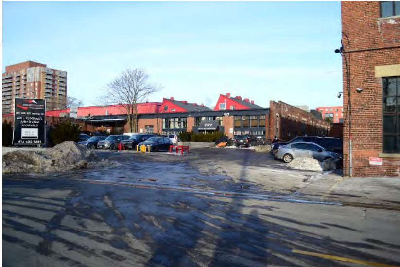
Figure 1 - Entrance to the subject site from Sterling Road, looking east, showing the former Moloney Electric building at 213-219 Sterling Road to the right.
