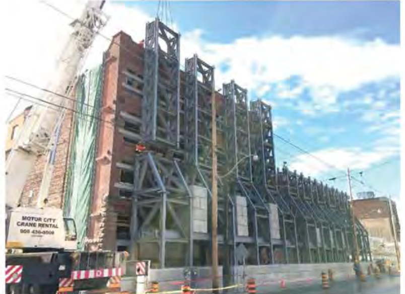
511-529 King St W – Exterior
