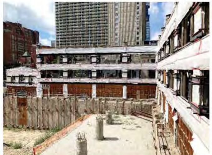
Internal looking west from Gerrard St east entrance
