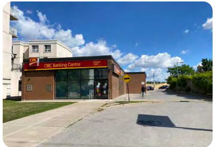
CIBC Banking Centre at 2340 Finch Avenue West, looking north
