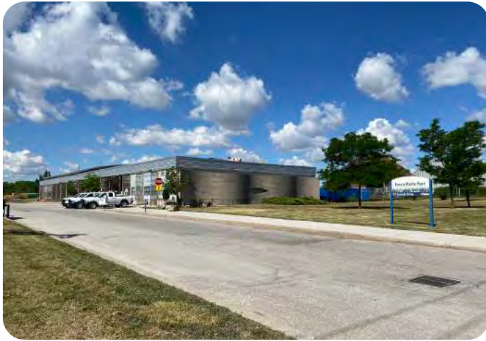
Emery Parks Yard at 27 Toryork Drive, looking southwest
