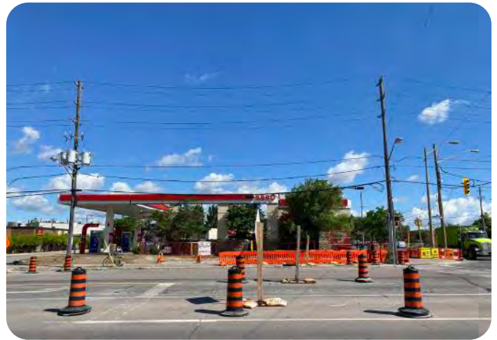
Gas Station at 3514 Weston Road, looking north
