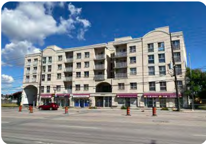
5-Storey Residential Mixed-Use Building at 2350 Finch Avenue West, looking northwest
