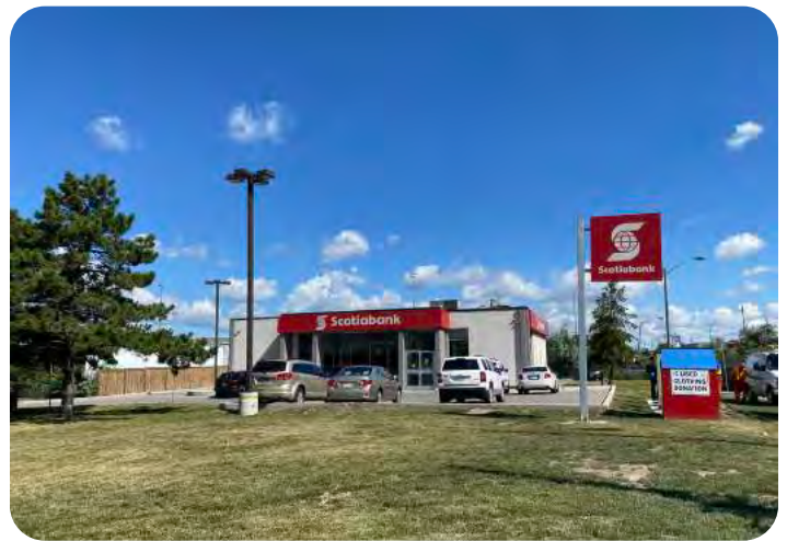
Scotiabank at 2 Toryork Drive, looking north
