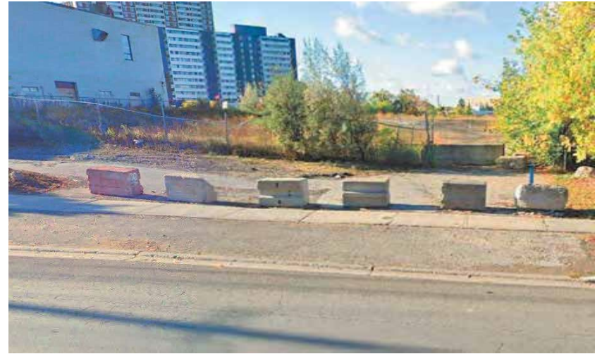
Figure 2c: Toryork Drive looking south at the site
