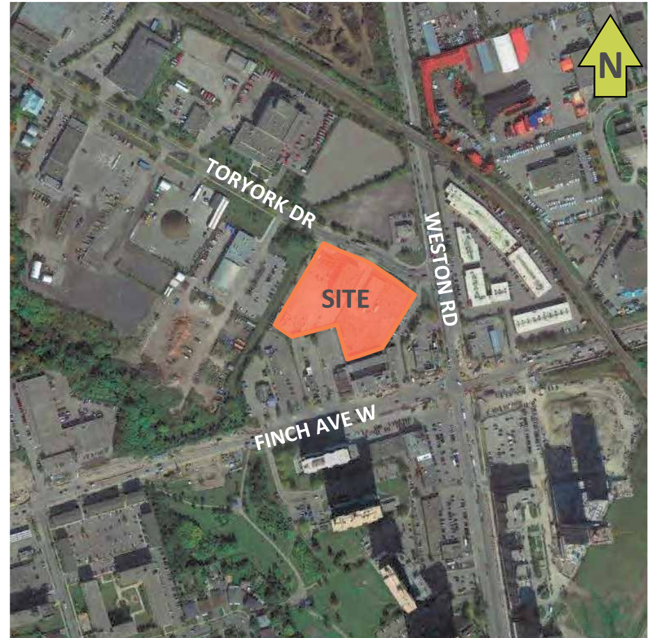
Figure 1: Aerial view of existing site & surroundings Credit: Google Earth Pro, dated 10/4/2022
