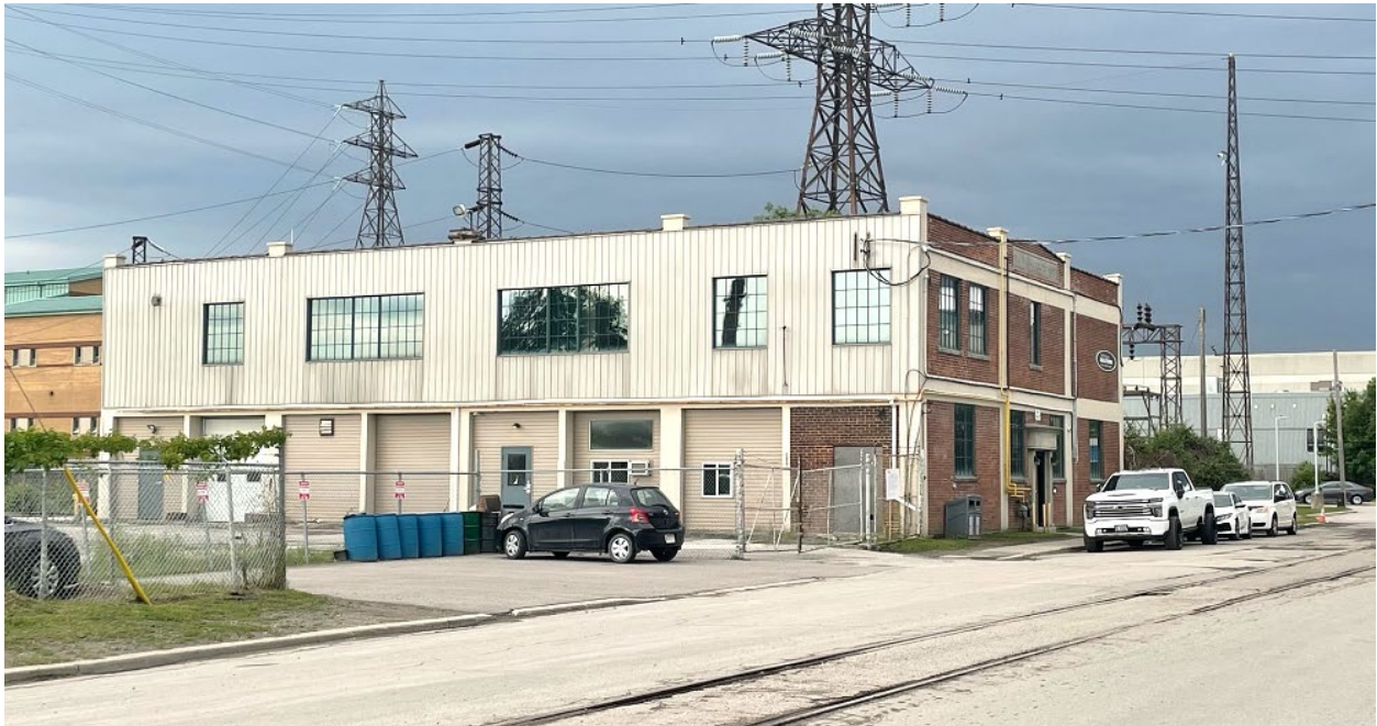
Figure 15. Context view looking west. Heritage Planning, 2023.
