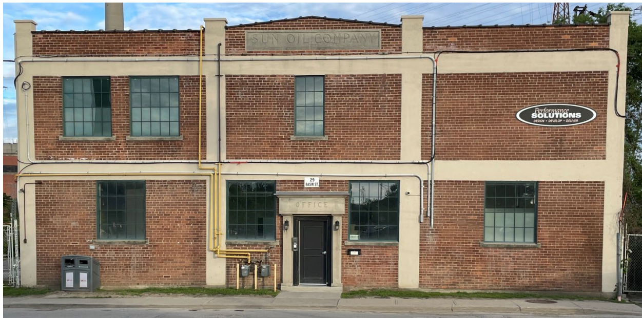
Sun Oil Company Building, front (north) elevation. Heritage Planning, 2023
