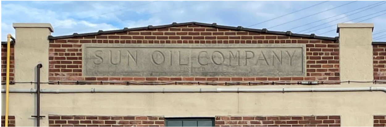
Figure 10. Sun Oil Company Building, cast stone entablature. Heritage Planning, 2023.
