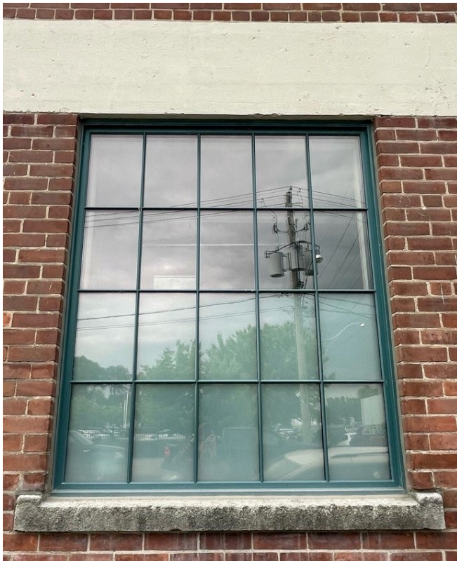
Figure 13. Sun Oil Company Building, replacement window. Heritage Planning, 2023.
