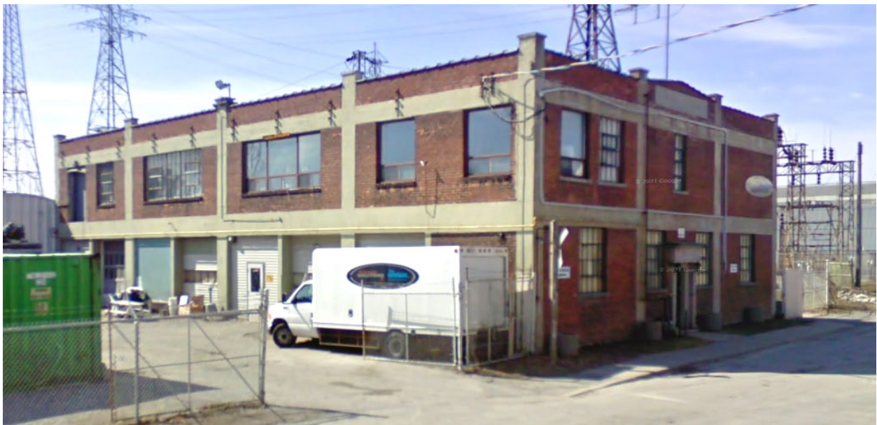
Figure 8. Sun Oil Company Building in 2009 prior to the recladding of the east elevation and 2019 masonry restoration and window replacement work. Google Maps.
