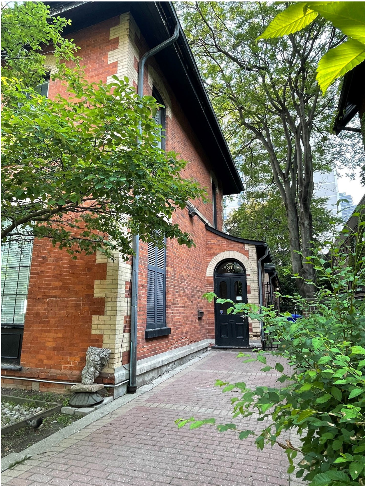
Figure 18: West elevation of 37 Maitland Street, 2023 (City of Toronto Heritage Planning)
