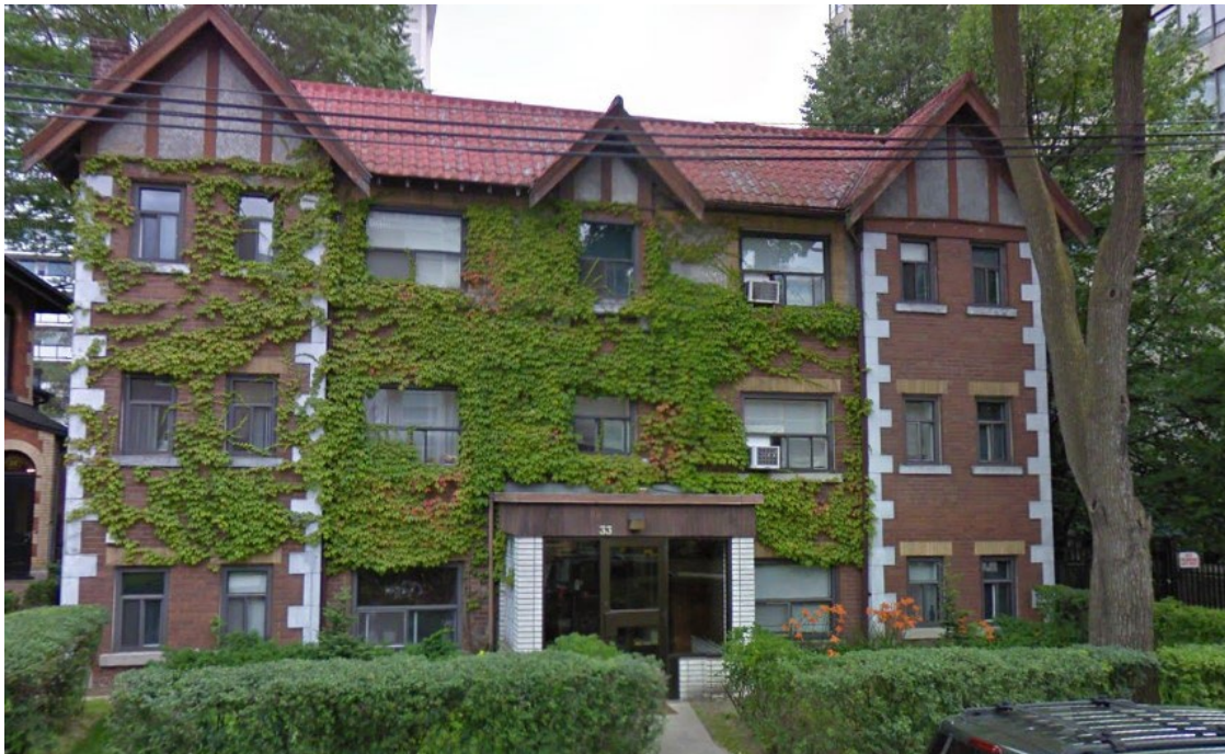
Figure 12: View showing original half-timbered gables, open eaves with exposed rafters, stucco-clad third storey, and metal Spanish tile roofing, 2009 (Google Maps)
