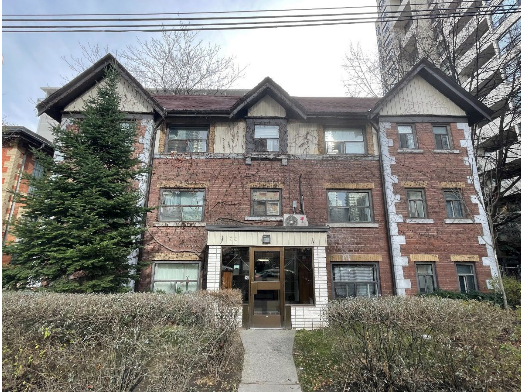
Figure 5: Front (north) elevation of 33 Maitland Street, 2023 (City of Toronto Heritage Planning)
