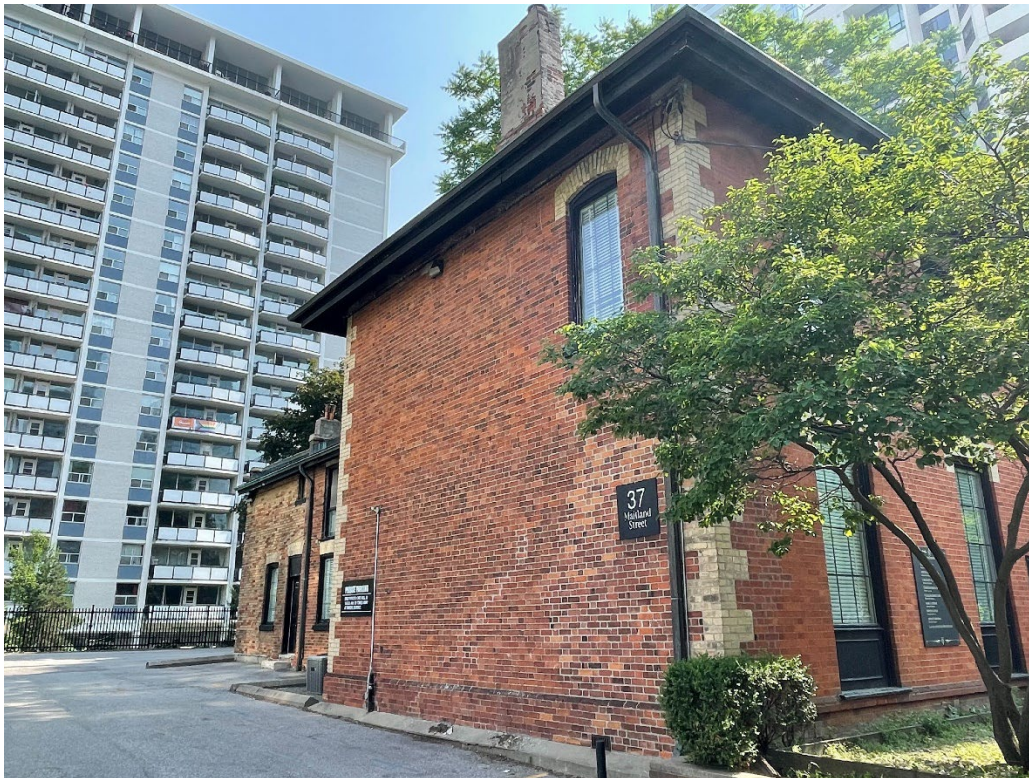
Figure 15: East elevation of 37 Maitland Street, 2023 (City of Toronto Heritage Planning)
