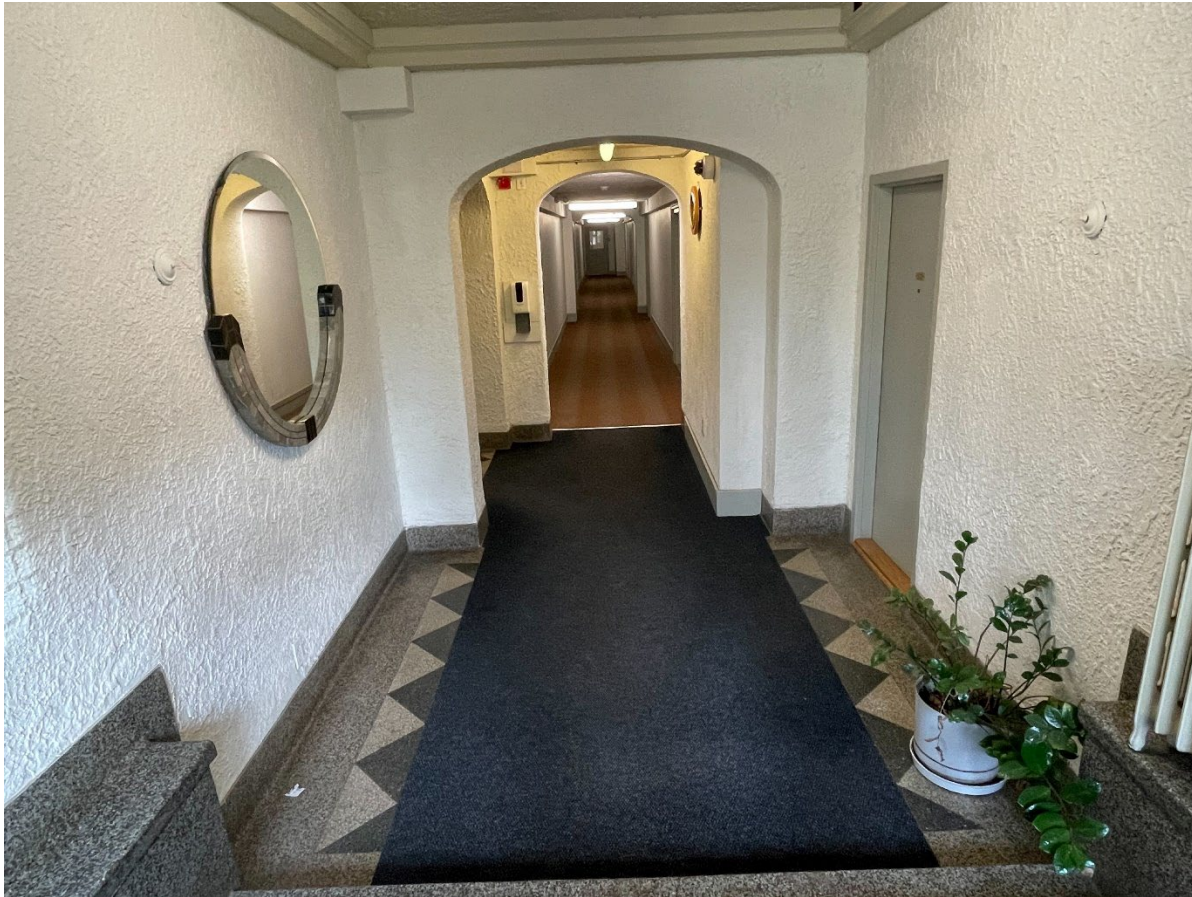
Figure 8: Interior view of foyer and ground floor corridors of 33 Maitland Street, 2023 (City of Toronto Heritage Planning)
