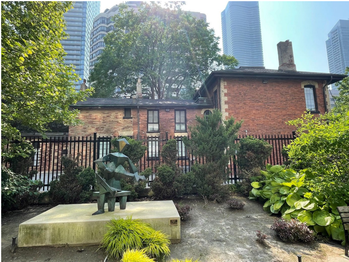
Figure 16: East elevation of 37 Maitland Street, 2023 (City of Toronto Heritage Planning)
