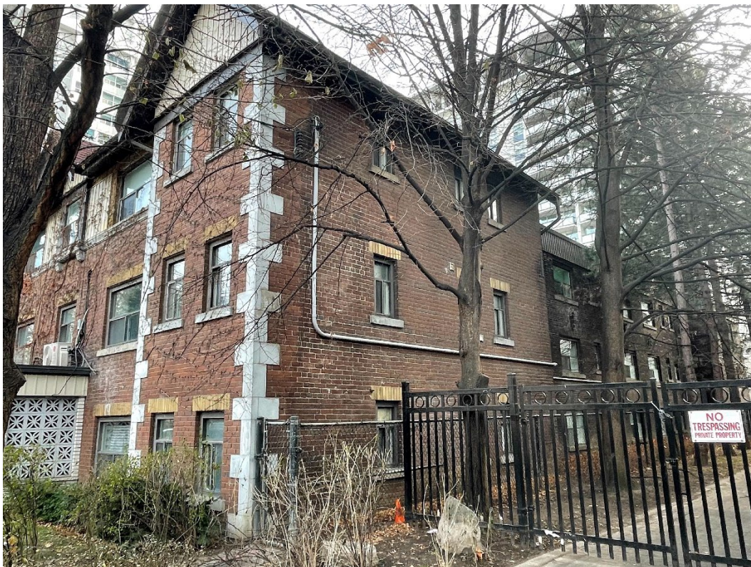
Figure 6: West elevation of 33 Maitland Street, 2023 (City of Toronto Heritage Planning)
