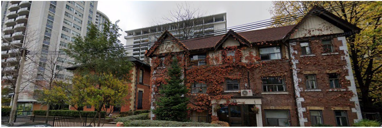
Figure 9: Contextual view from northwest showing 33 Maitland Street (right) and 37 Maitland Street (left), October 2020 (Google Maps)
