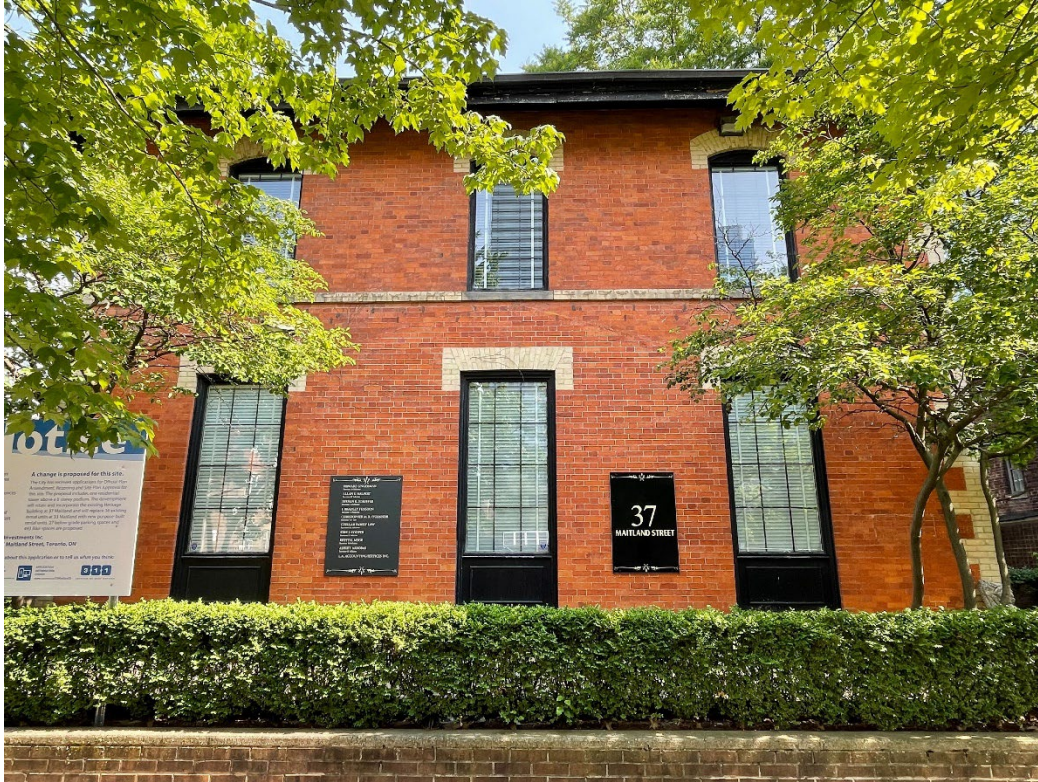
Figure 14: Main (north) elevation of 37 Maitland Street, 2023 (City of Toronto Heritage Planning)
