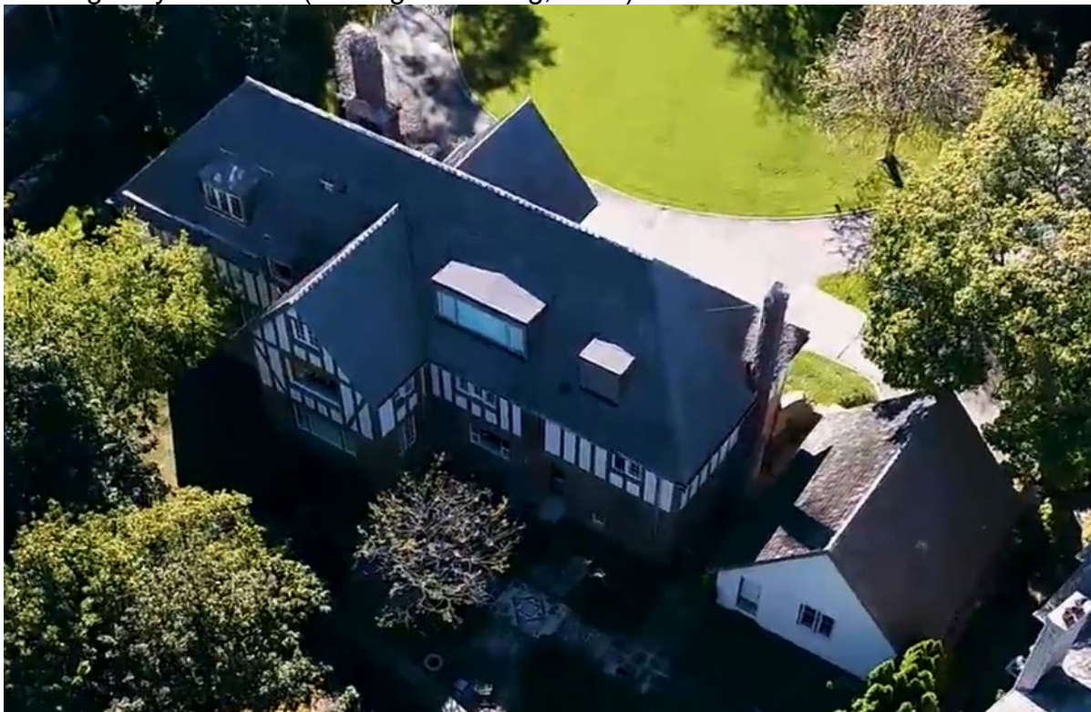
Contextual photo showing the existing detached garage at 35 Kingsway Crescent ( www.birdhousemedia.ca )
