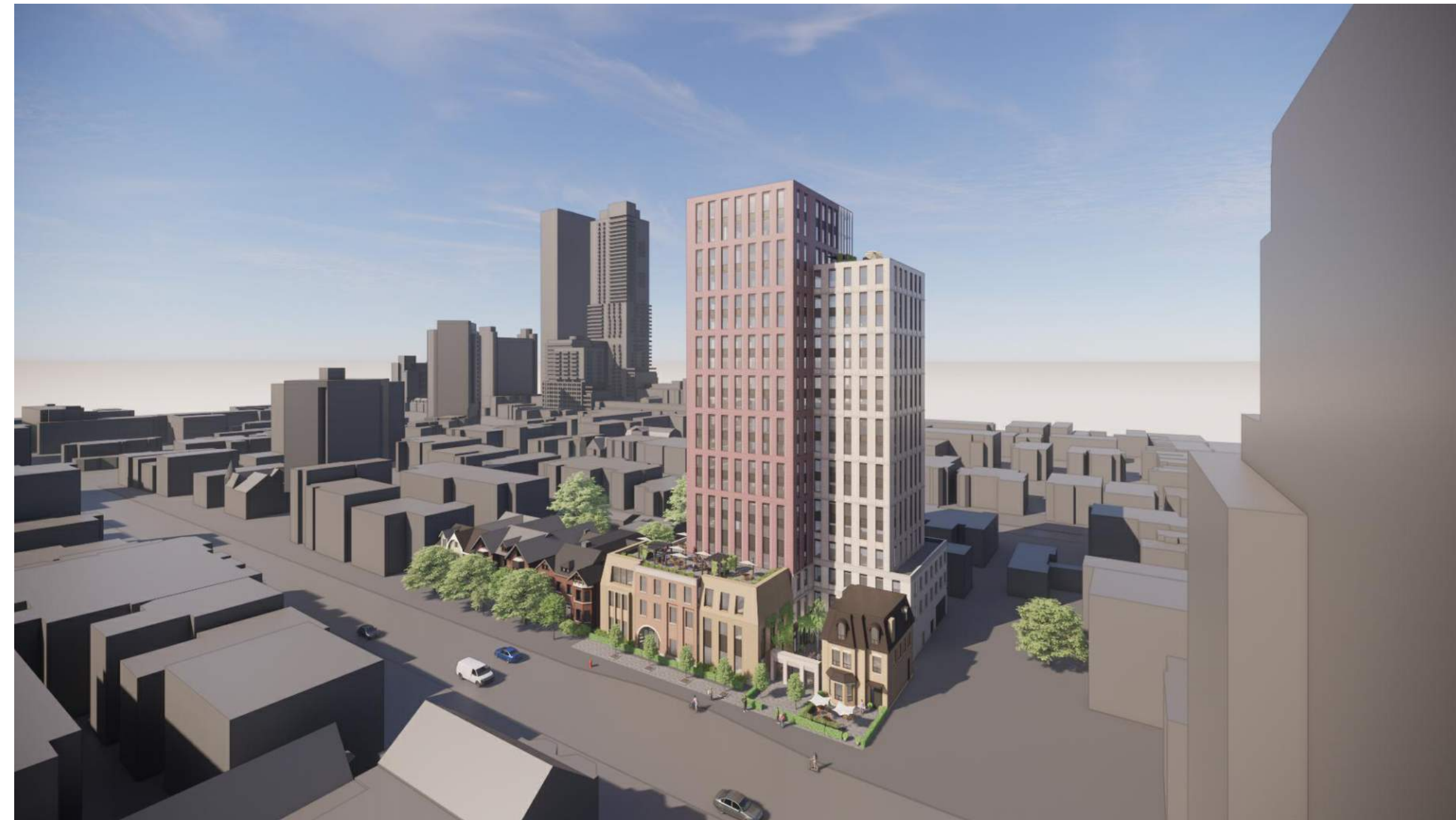
NORTH EAST AERIAL VIEW FROM SHERBOURNE ST.
