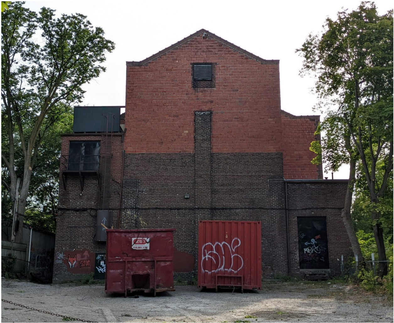
Figure 5. East elevation of 551 Mount Pleasant Road (Heritage Planning, 2022).
