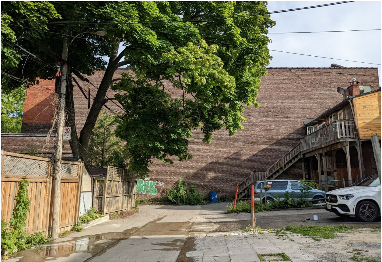
Figure 4. North elevation of 551 Mount Pleasant Road (Heritage Planning, 2022).
