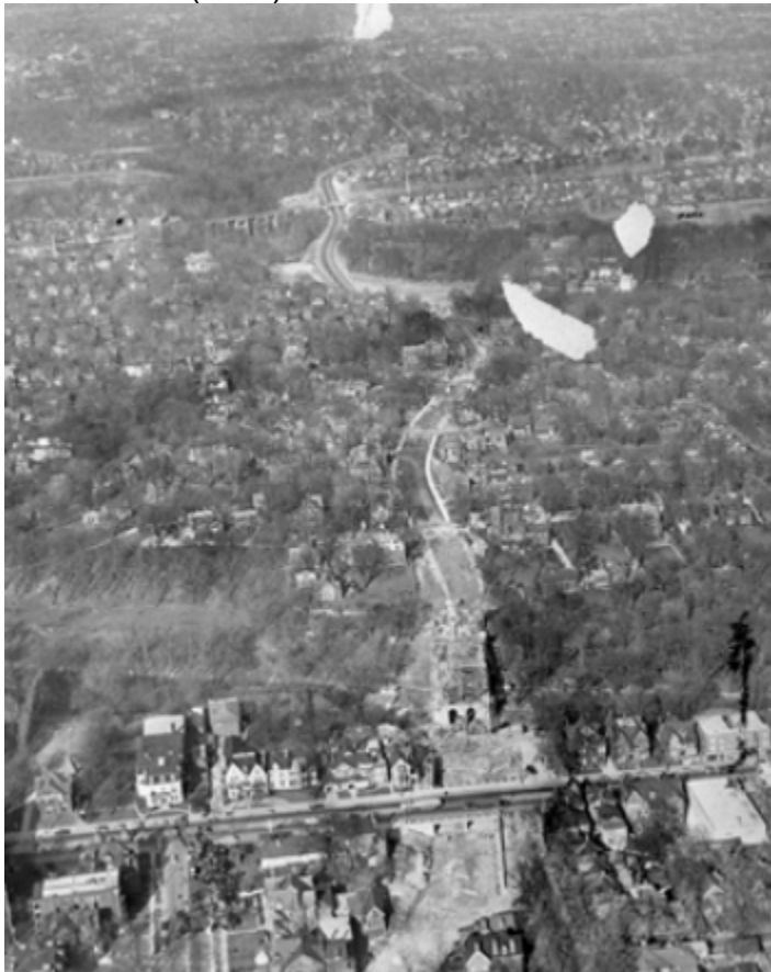
Image 9. 1946 aerial photograph looking north from south of Bloor Street East at the Clifton Road Extension under construction. (Toronto Public Library)
