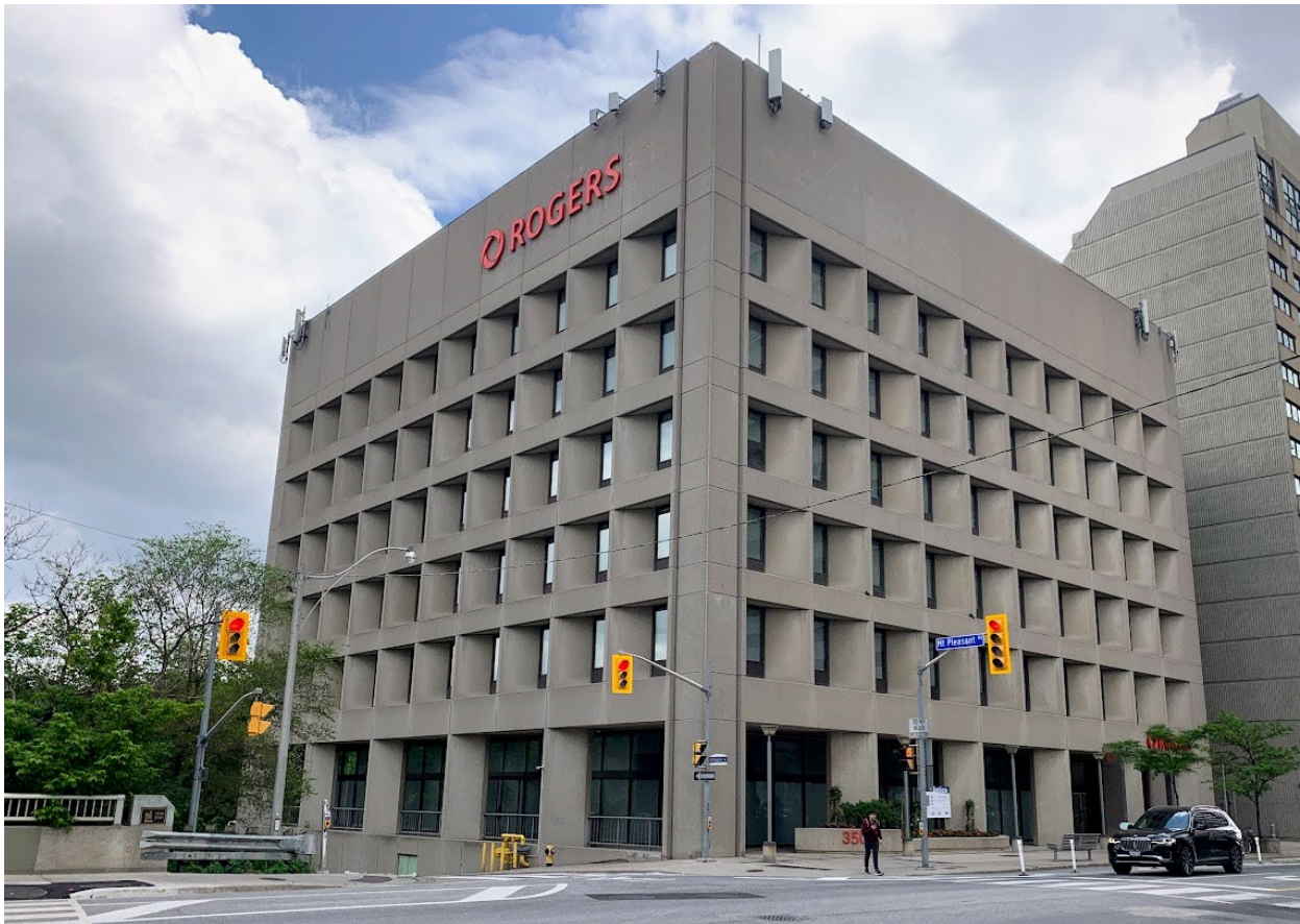
Above: Current photo looking northeast from Bloor Street East and showing the south and west elevations of 350 Bloor Street East (Heritage Planning, 2023)
