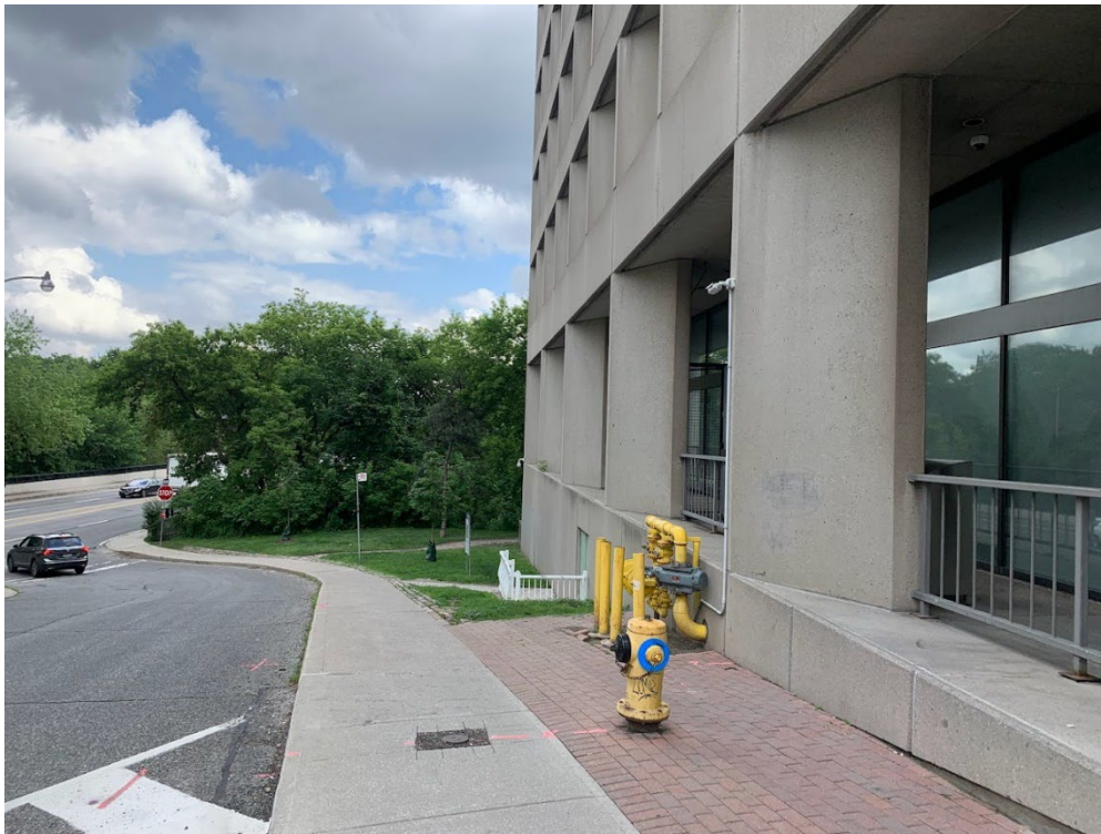
Image 42. Current photograph looking north and showing the transition of the pedestrian colonnade to a colonnaded terrace on the west elevation.
