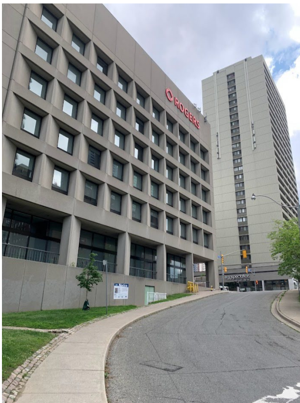
Image 43. Current photograph looking south and showing the colonnaded terrace on the west elevation and the steep grade change of the site. (Heritage Planning, 2023)
