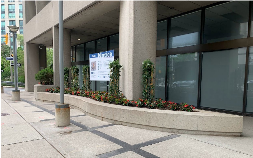
Image 39. Current photograph showing the undulating 1990s concrete planter added to the base of several perimeter columns on the south elevation (Heritage Planning, 2023)
