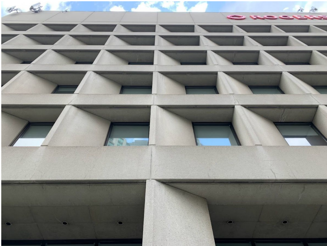
Image 35. Current photograph looking up at the pre-cast concrete panels and openings on the south elevation (Heritage Planning, 2023)
