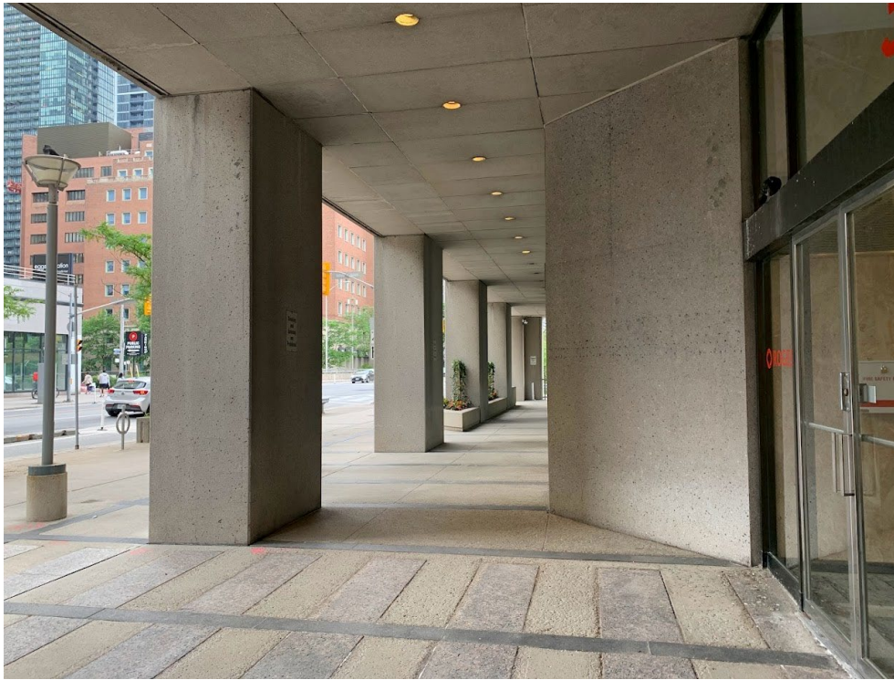
Image 40. Current photograph looking west along the pedestrian colonnade from the main entrance (Heritage Planning, 2023)
