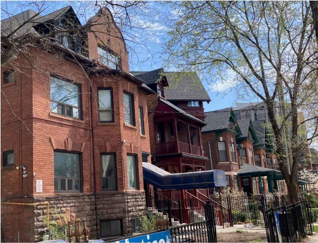
Figure 13: 409 Huron Street (left) within streetscape context, 2023 (Heritage Planning).
