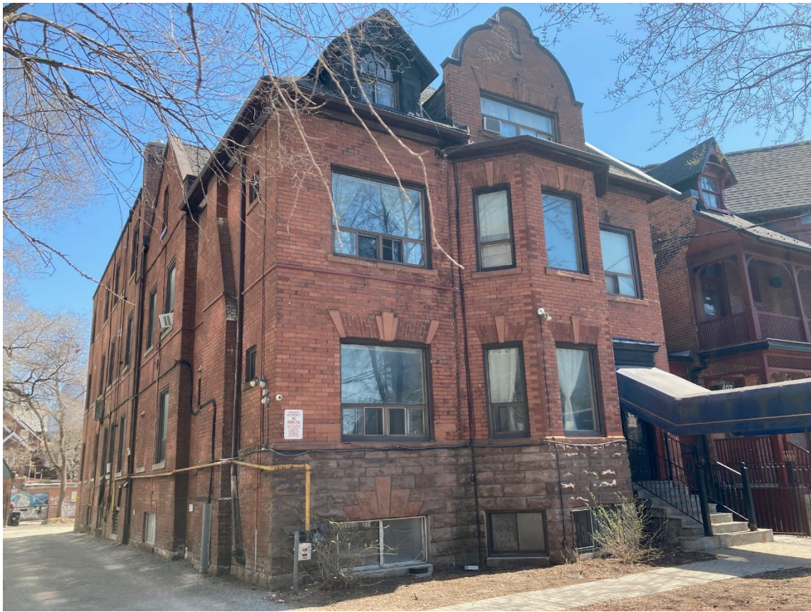
Figure 11: West and north elevations, 2023 (Heritage Planning).
