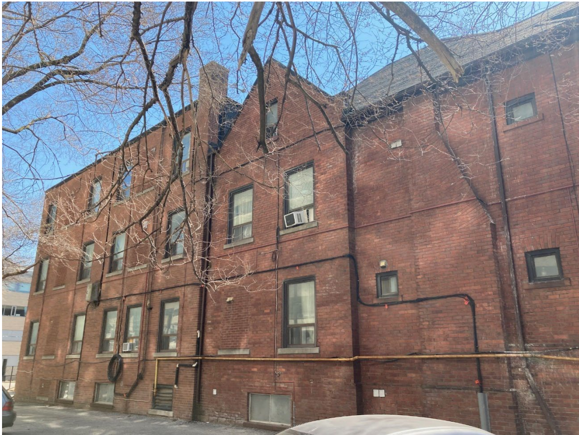
Figure 12: North elevation showing addition at rear, 2023 (Heritage Planning).
