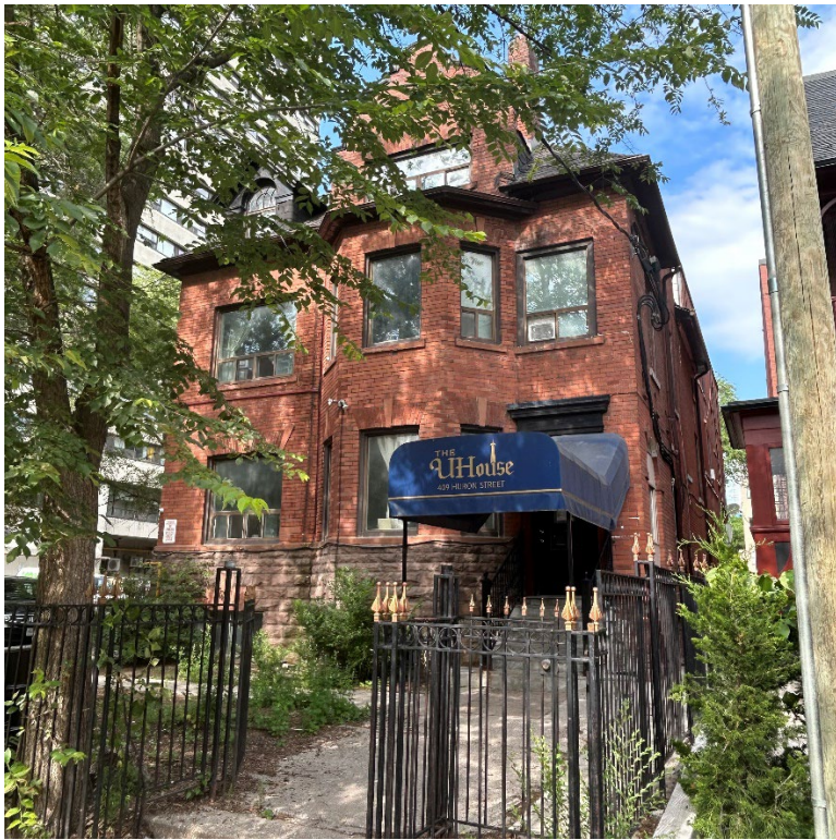
Figure 9: 409 Huron Street, primary (west) elevation, 2023 (Heritage Planning).
