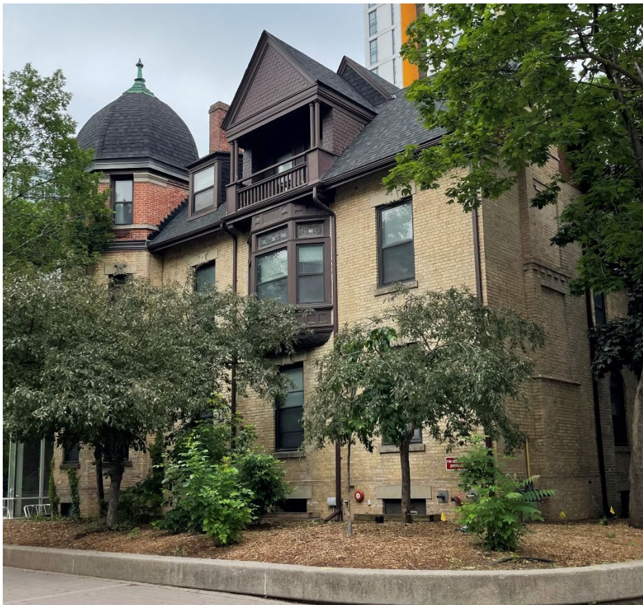
Figure 21. 137 Bond Street north and west elevations (Heritage Planning, 2023).
