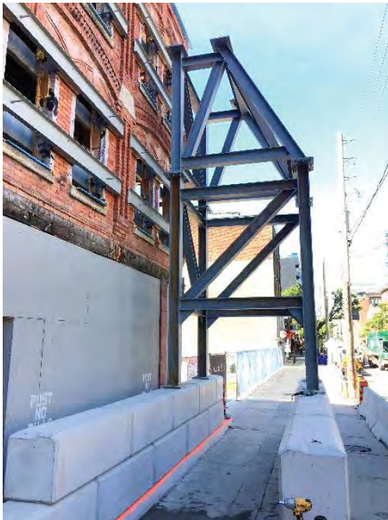
511-529 King St W – Pedestrian walkway
