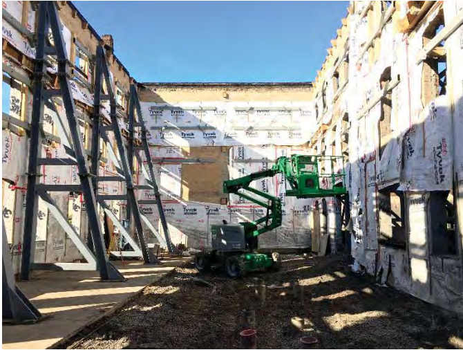
495 King St W – Interior, south elevation
