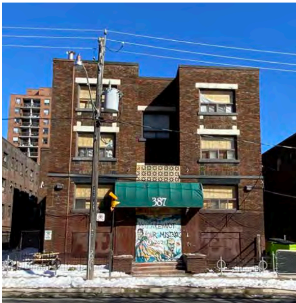
Fig.40: Overall view of the west façade.
