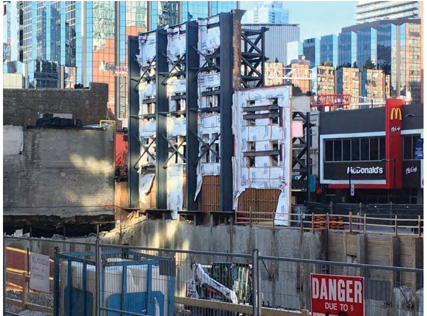
Internal four-and-a-half storey vertical stiffening beams connected to shoring piles
