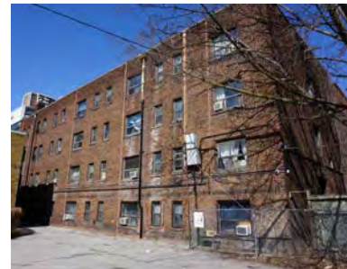
Fig.2: View of the south and east façade.
