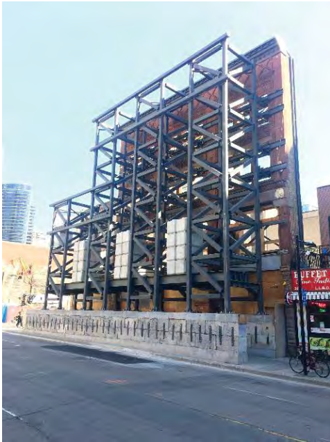
Exterior four-and-a-half storey
