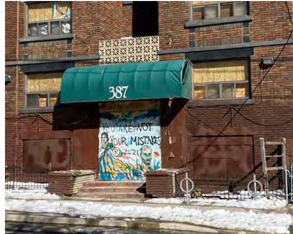
Fig.42: Condition at grade, west façade.
