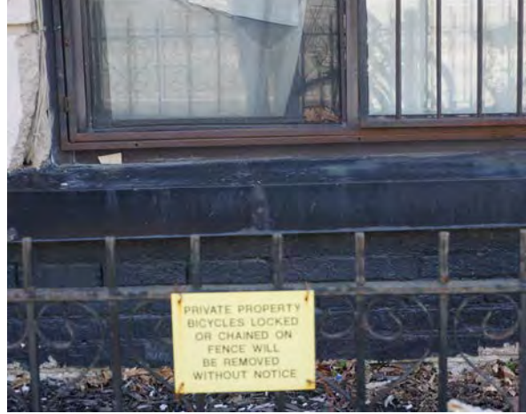
Fig.19: Example of sill flashing condition with warping and dents on the west façade.
