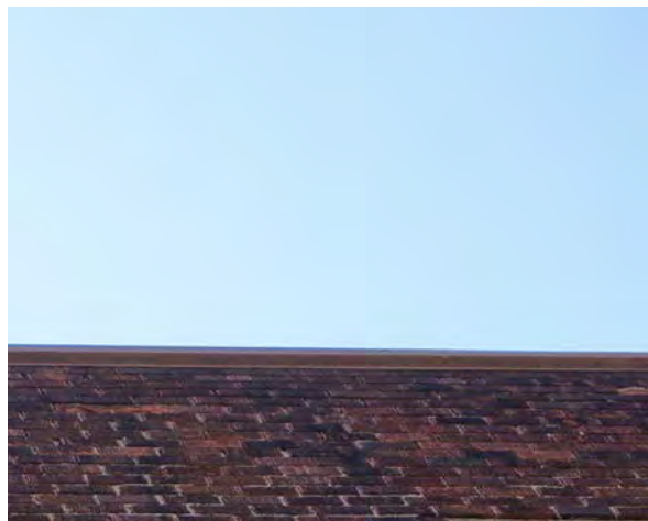
Fig.39: Detail of metal roof flashing on the north façade.
