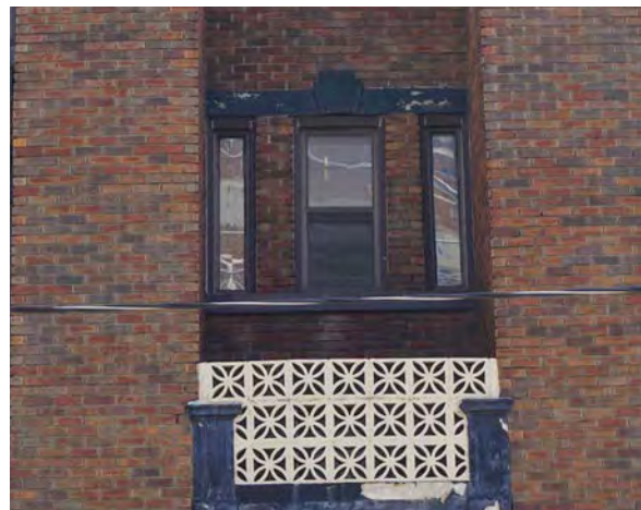
Fig.6: Detail of the second storey light well on the west façade.
