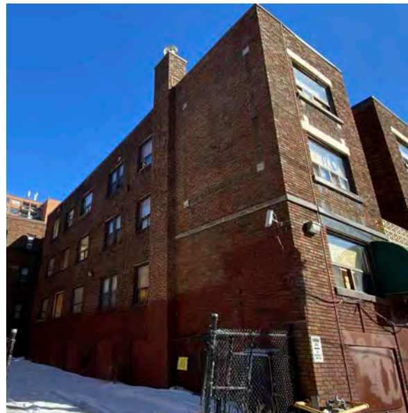
Fig.41: Overall view of the north façade.
