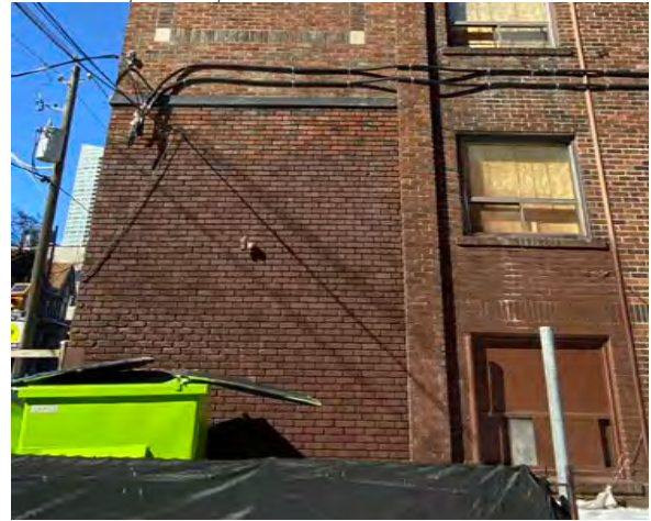
Fig.52: Painted masonry at lower storeys of south façade.
