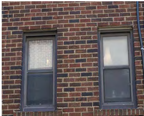
Fig.38: Detail of the windows at the north façade.
