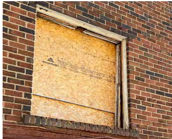
Fig.56: Traces of wood window in opening, north façade.
