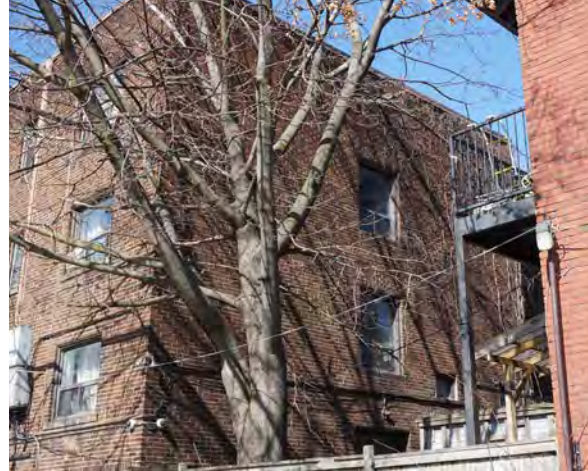
Fig.31: View of the masonry on the east façade.
