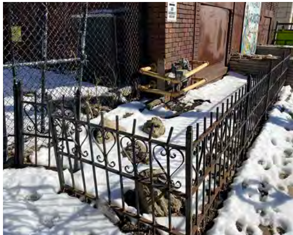
Fig.61: Condition of wrought iron fencing, west façade.
