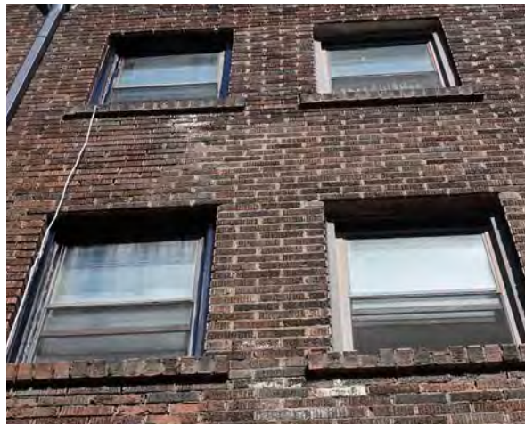
Fig.29: Example of windows along the south façade.
