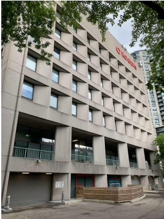
View showing the north elevation with the colonnaded pedestrian terrace and exposed lower level containing the entrance to the second lower level parking garage. (Heritage Planning, 2023)
