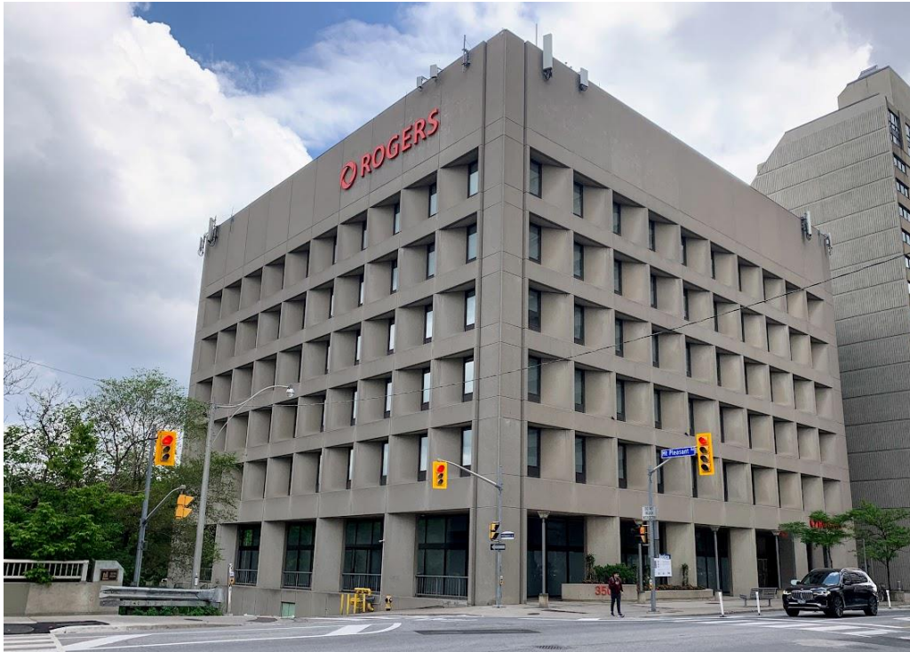
View looking northeast from Bloor Street East and showing the south and west elevations of 350 Bloor Street East (Heritage Planning, 2023)
