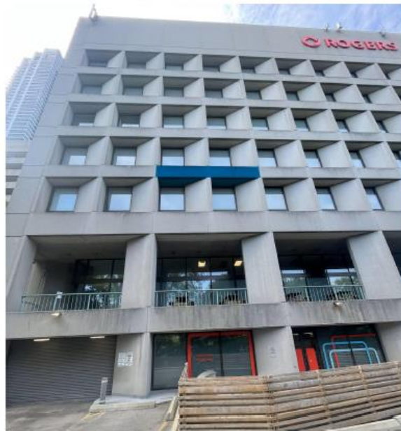
North Elevation – Site Photo
